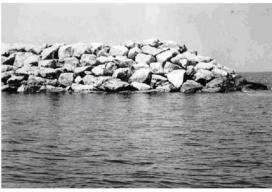
Figure VI-4-3. Selective placement (USACE, COASTAL ENGINEERING MANUAL)
