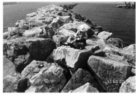
Figure VI-4-2. Random placement (USACE, COASTAL ENGINEERING MANUAL)
