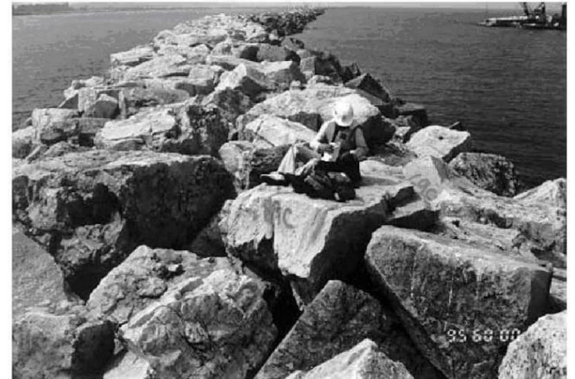
**Figure VI-4-2. Random placement** (USACE, COASTAL ENGINEERING MANUAL)
