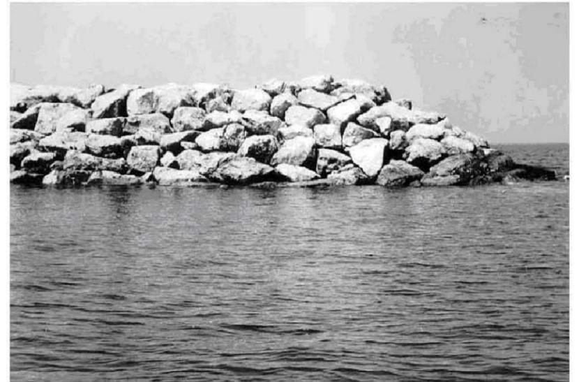
**Figure VI-4-3. Selective placement** (USACE, COASTAL ENGINEERING MANUAL)
