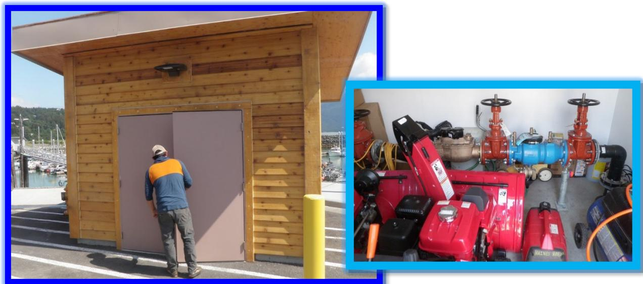
Figure 4.2: New Harbor Improvements — RPZ Assembly, 2022 Sanitary Survey
