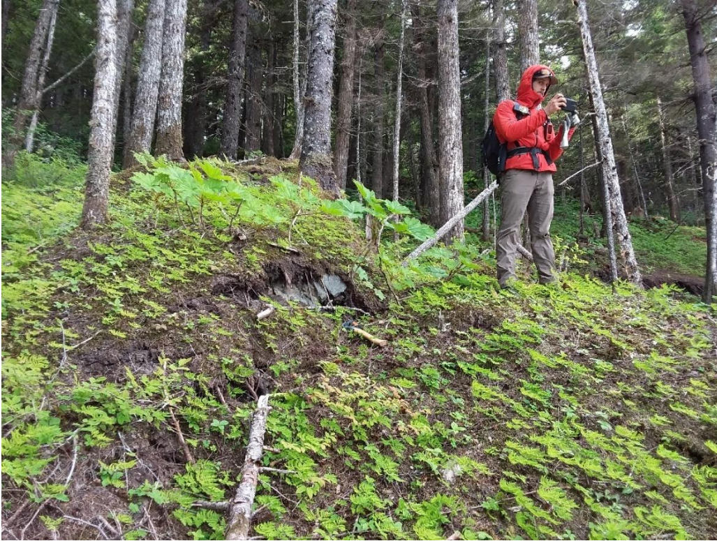
A: Looking southwest along a tension crack that parallels the eastern lateral scarp (i.e. 035-040° azimuth).
