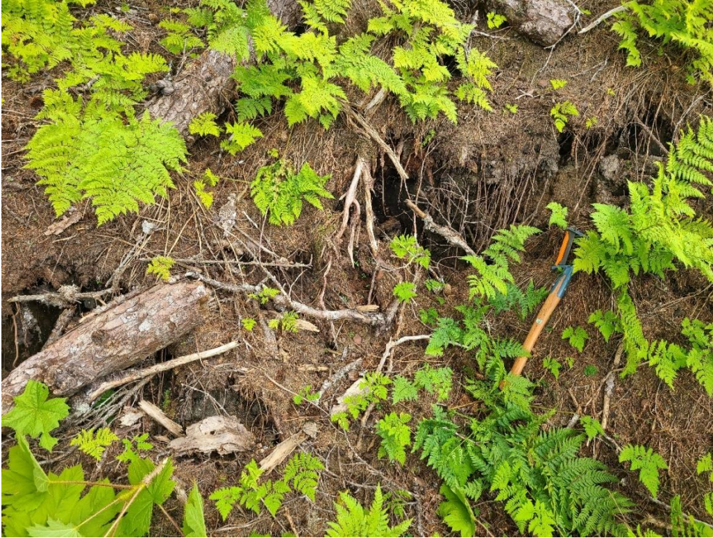
A: Looking south at a tension crack adjacent to the eastern lateral scarp near elevation 745 feet.
