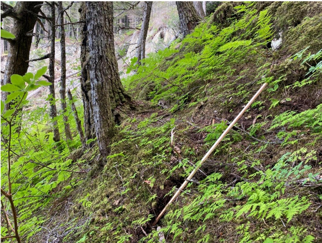
B: Looking northeast along the west tension crack.
