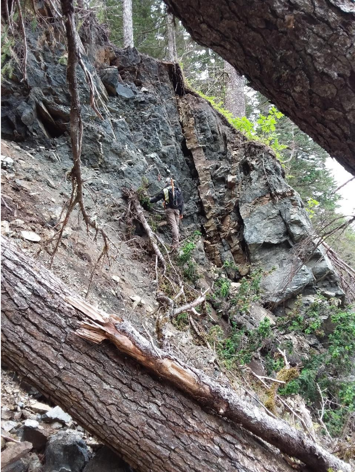
Looking west at the central portion of the headscarp with layered ultramafic rock exposures.
