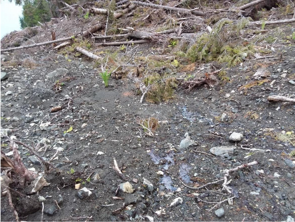
A: Looking south at a seepage point above flow near the eastern side of the slide near elevation 280 feet.
