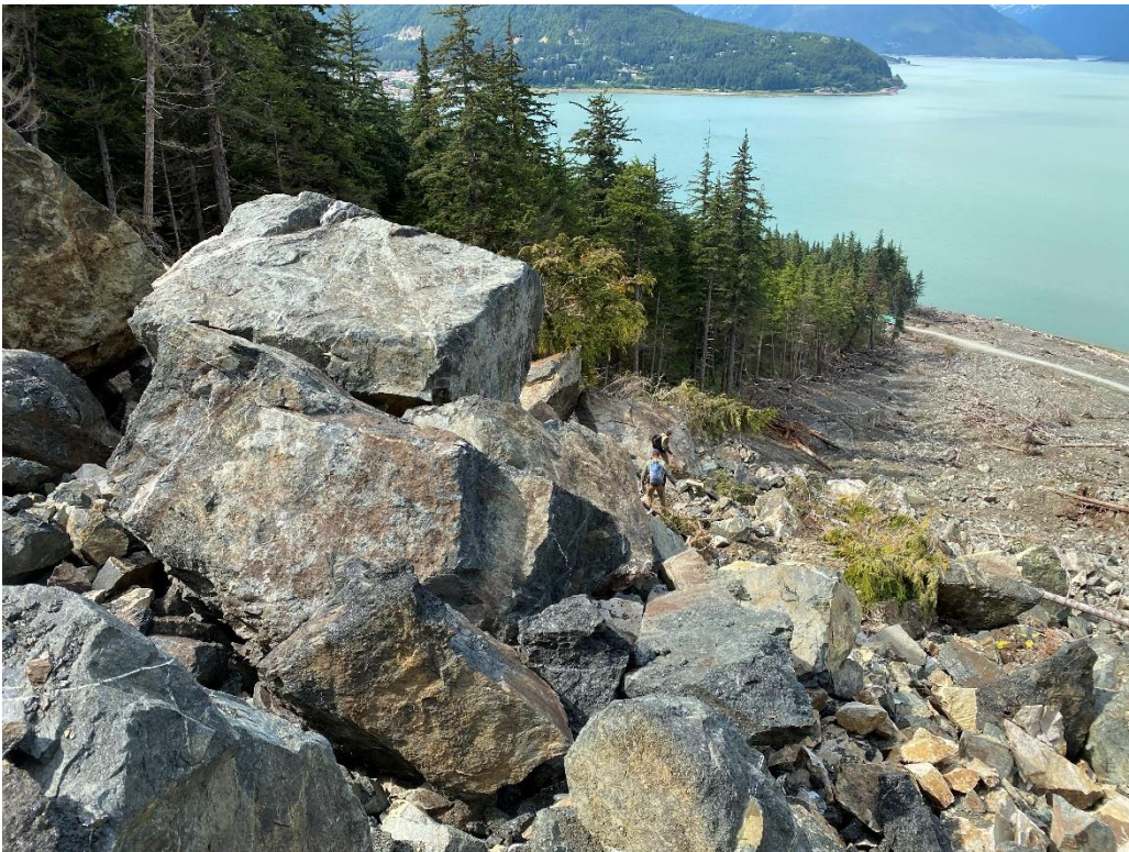
B: Looking northwest at the boulder field in the main body of the slide.
