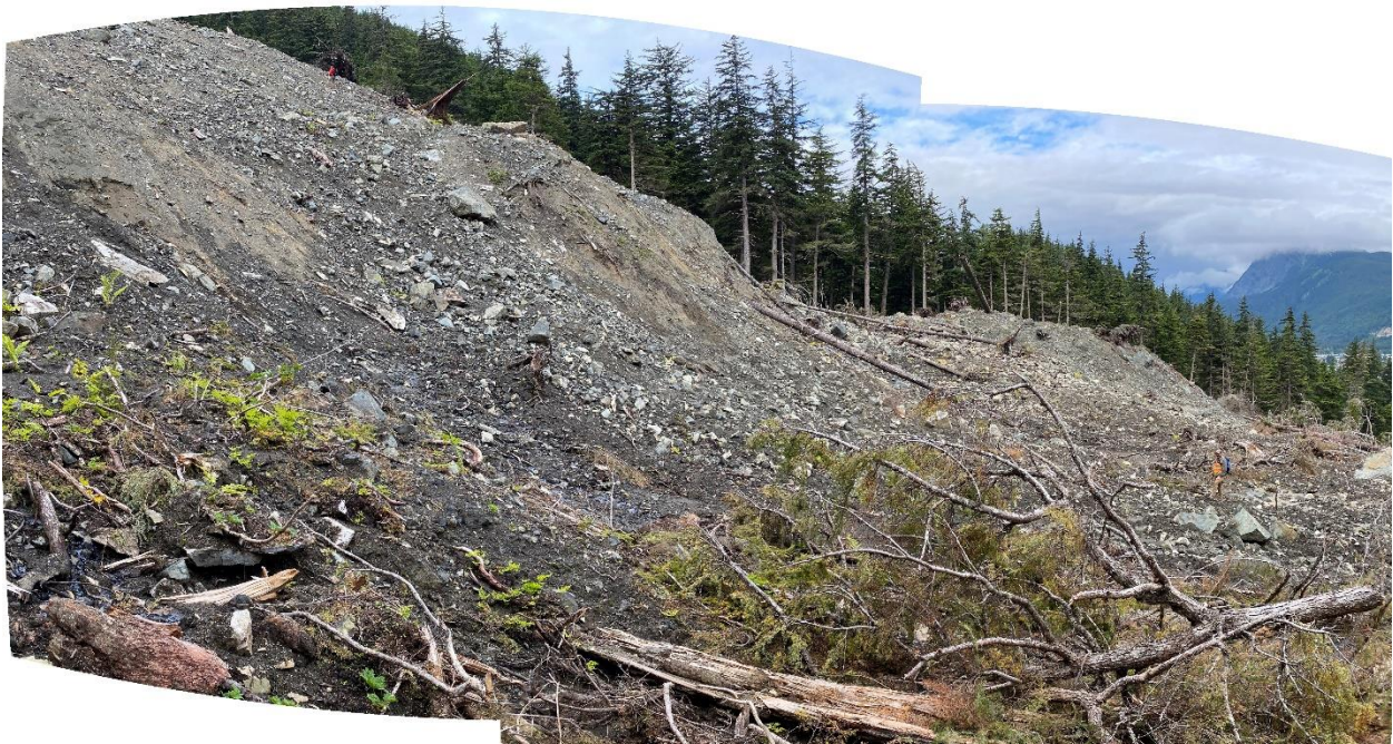
Looking west at scoured soil (middle ground center and left) between gravel and boulder debris deposits on the slope above the lower Mt. Riley Road extension bench.
