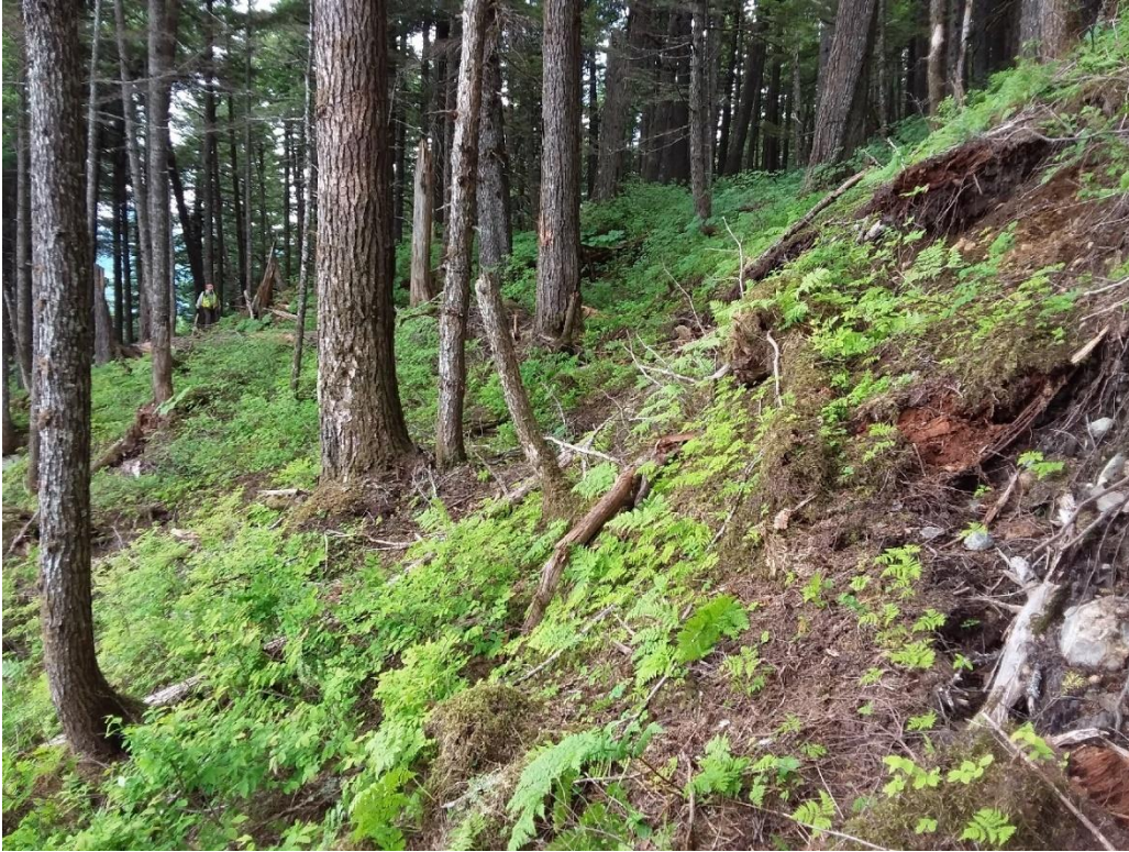
A: Tension, down drop and cavities along the eastern tension crack.
