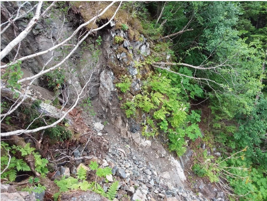
B: Looking west at the western lateral scarp rock exposures.
