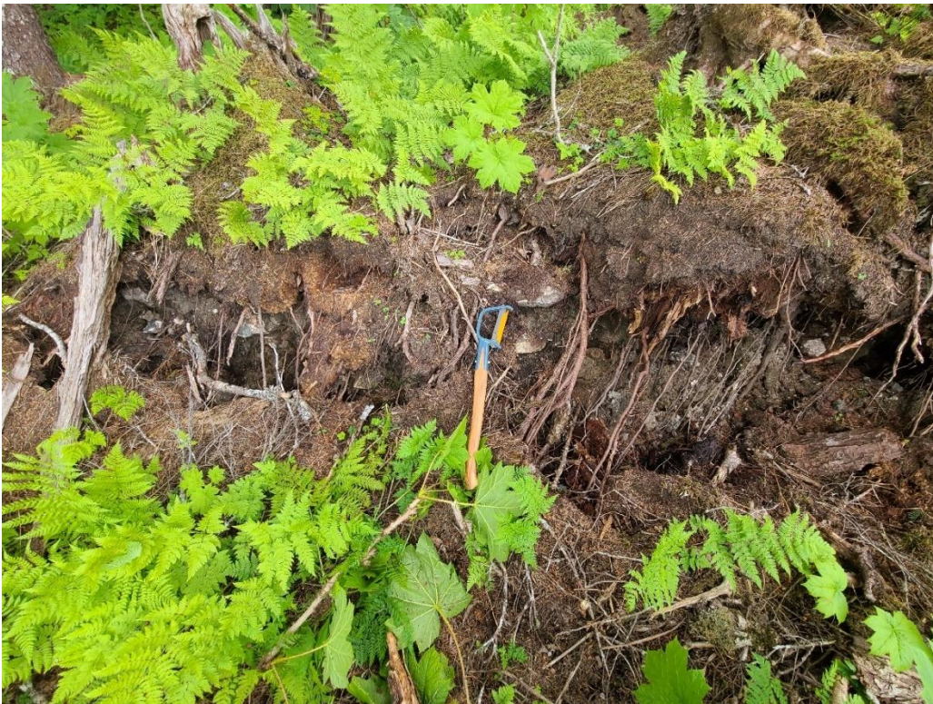
B: Looking south at a tension crack adjacent to the eastern lateral scarp near elevation 745 feet.
