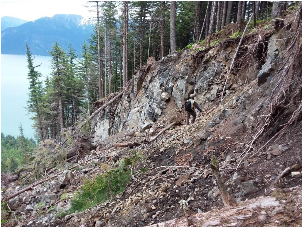
B: Looking northeast at the eastern lateral scarp rock exposures.
