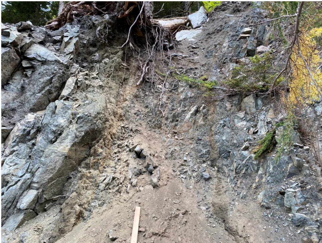
B: 4-foot wide fault near parallel to layered rock at elev. ~810 ft in eastern lateral scarp.
