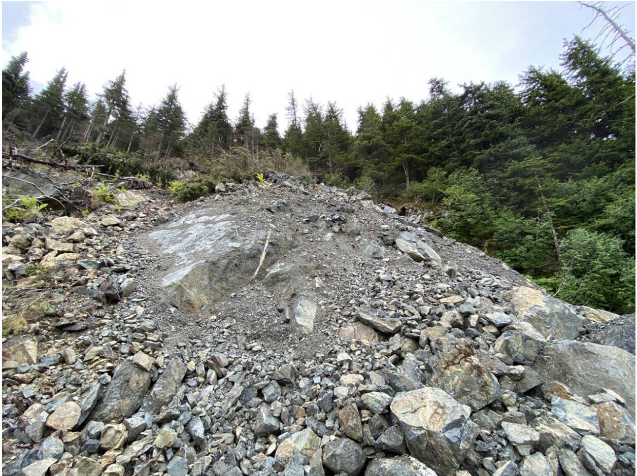
Looking south at a dilated slump block adjacent to the western lateral scarp near elevation 670 feet.
