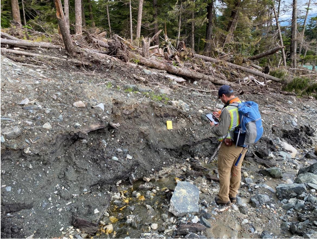
A: Looking west at exposed slide debris and pre-existing ground in the western lateral extents on the lower portion of the slide.
