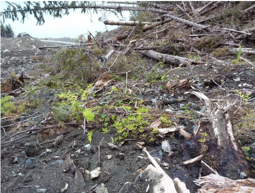
B: Looking north at a seepage point above flow near the eastern side of the slide near elevation 280 feet.
