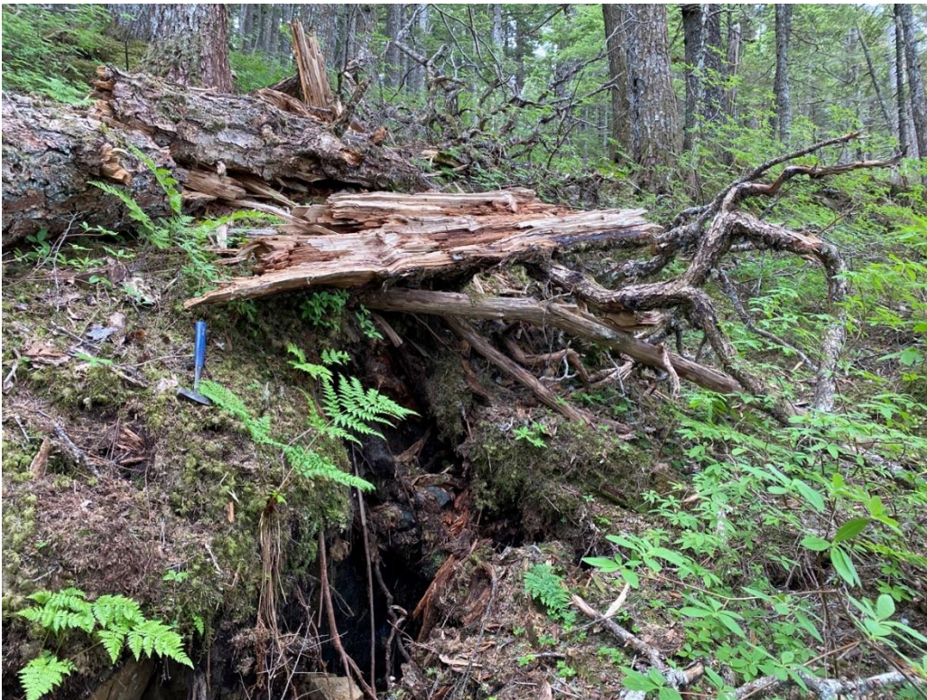
B: Looking southwest along the eastern tension crack, approximately 160 feet from the headscarp.
