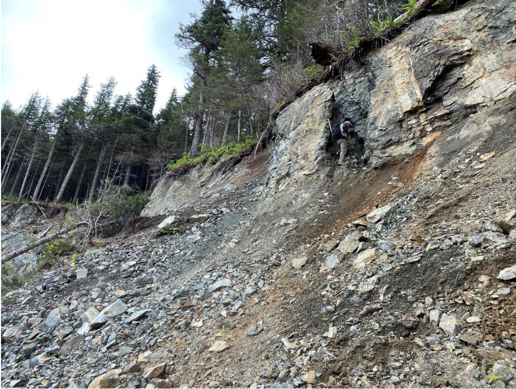
A: Looking southeast along the west central headscarp.
