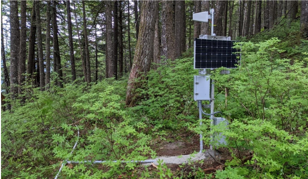
Photo 3: Datalogger post, enclosures, solar panel, and cellular antenna.
