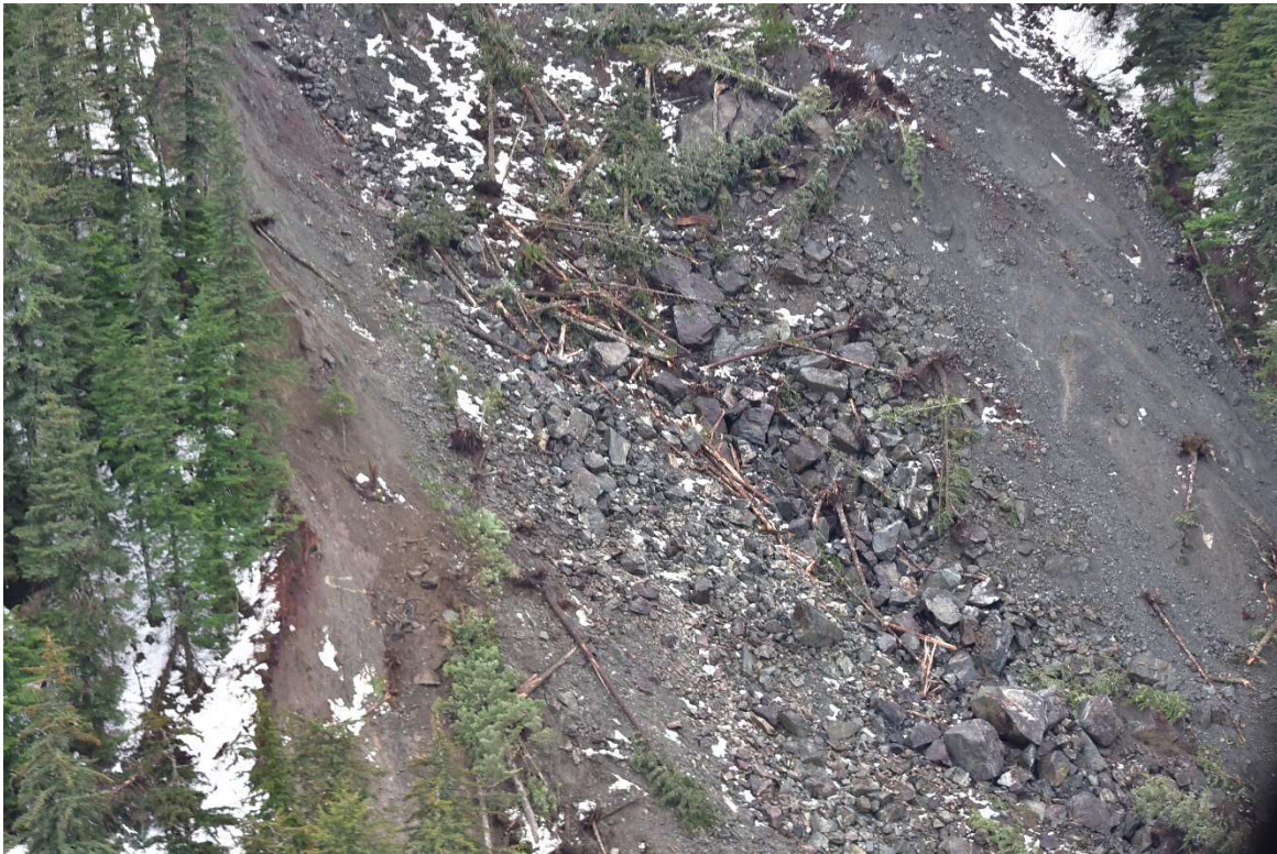
View looking south at landslide debris in upper portion of landslide (from Haines Avalanche Center, taken 12/8/2020).
