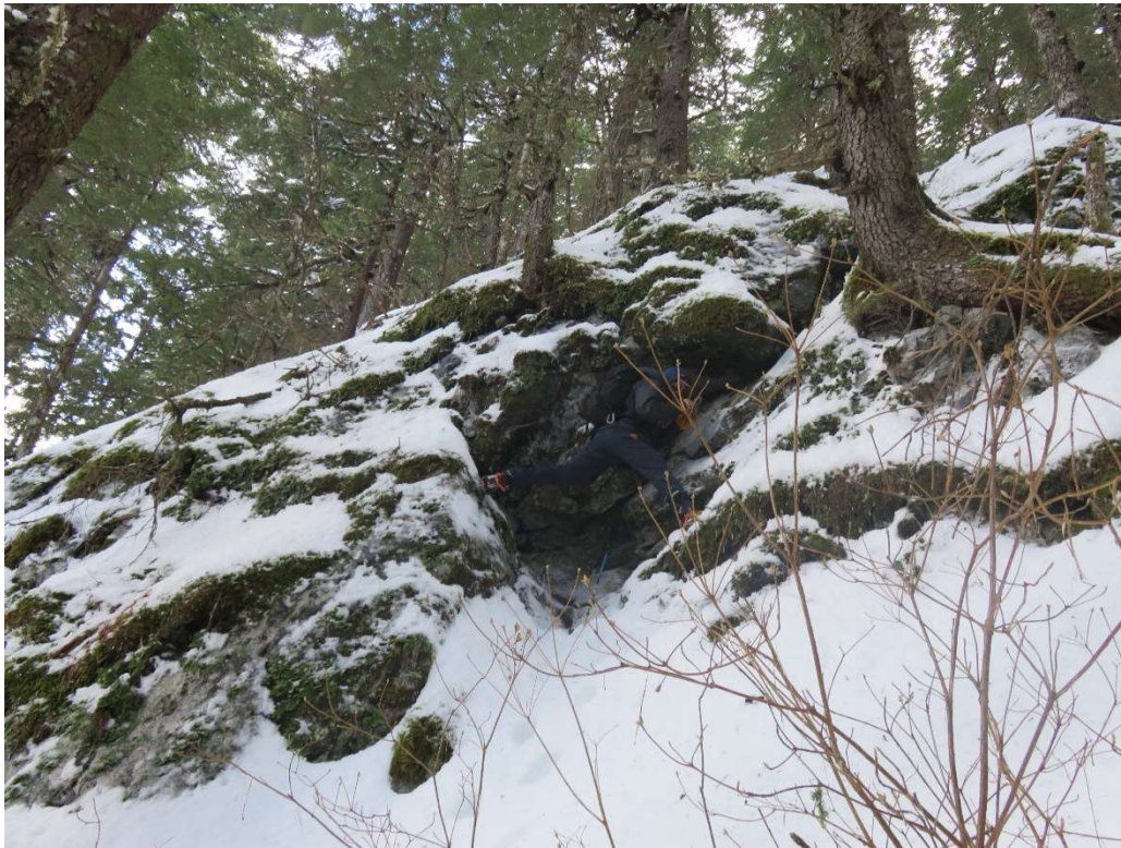
View looking southeast at rock outcrop on the western flank of the slide near elevation 550 feet (taken 2/23/2021).
