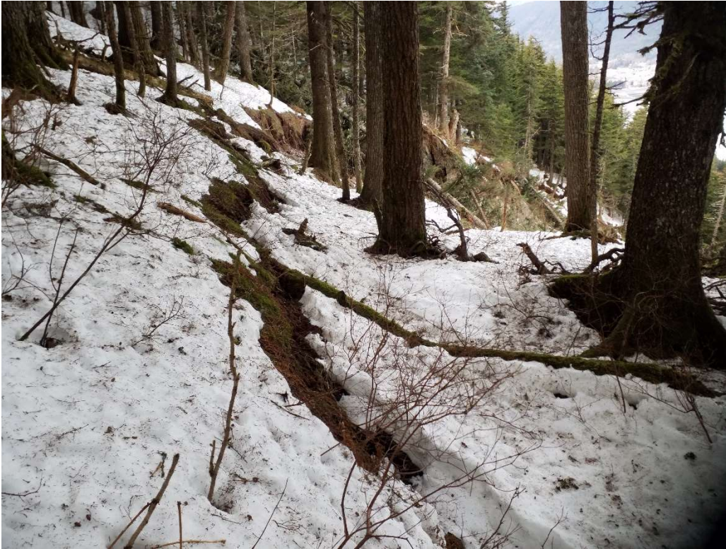
View looking west at easternmost extension of ground cracks east of the headscarp (from DGGS, taken 12/11/2020).
