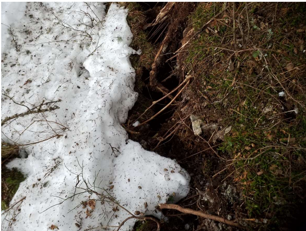
Close up view of ground cracks east of the headscarp (from DGGS, taken 12/11/2020).
