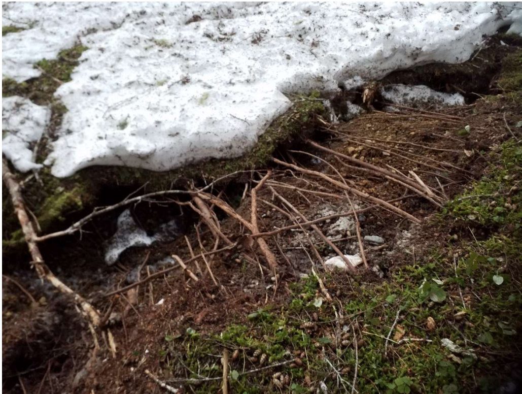
Close up view of ground cracks east of the headscarp (from DGGS, taken 12/11/2020).
