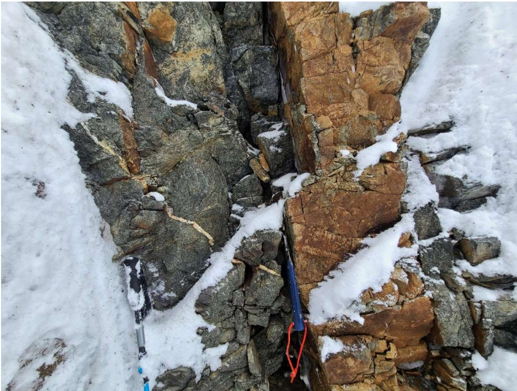
Close up view of rock exposed in the eastern portion of the headscarp. Note altered nature of the rock surface (taken 2/24/2021).
