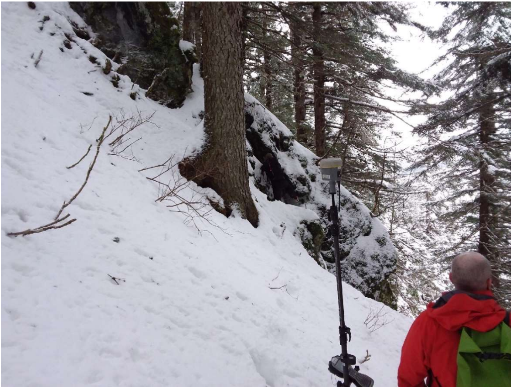
View looking east at the base of the eastern most prominent rock knob (east of the slide area; taken 2/25/2021).
