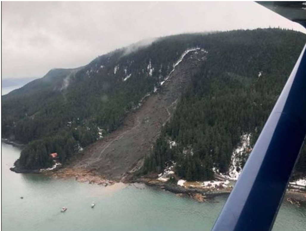
Aerial view looking southeast at landslide (from DGGS, taken 12/10/2020).
