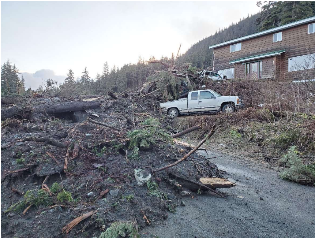
View looking southeast at landslide debris and damage to the Messano property (from Haines Avalanche Center, taken 12/9/2020).
