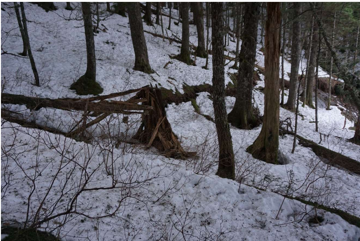
View looking southwest at easternmost extension of ground cracks east of the headscarp (from DGGS, taken 12/11/2020).
