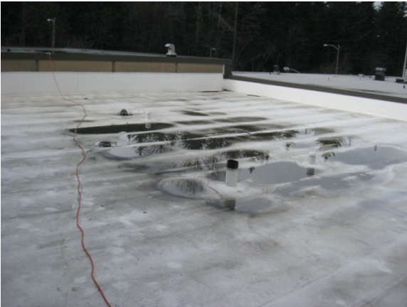
Overall view of Area 6.
