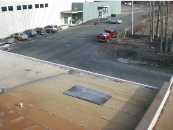
Overall view of Area 8.
