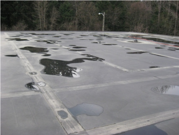
Overall view of Area 7.
