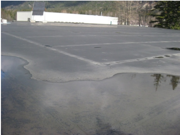
Overall view of gym roof.
