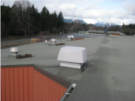
Pool roof looking west.
