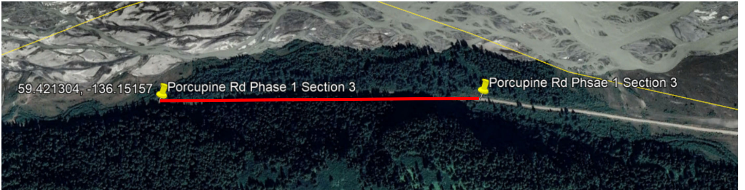
Google Earth – Showing the location of Phase 1, Section 3: Proximal the Chilkat River. The red line indicates the 0.6 miles of road work completed for Phase 1 Section 3.
