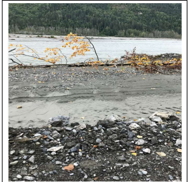
Site 9 GPS START: 59.41416, -136.08884 GPS END: 59.414363, -136.085552. Borrow Fill, 942.2222 CY of borrow fill, 636 FT long x 20 FT wide x 2 FT deep, high volume and high velocity surface water flooding scoured and washed out fill
