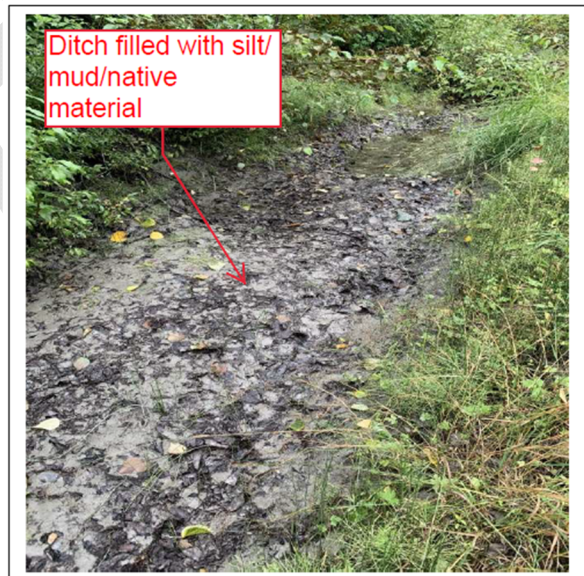
Site 2 GPS: 59.412354, -136.029592: Ditches, 7,626.6667 CY of native material drainage canals, 34,320 FT long x 3 FT wide x 2 FT deep, high volume and high velocity surface water flooding scoured and washed out ditches.
