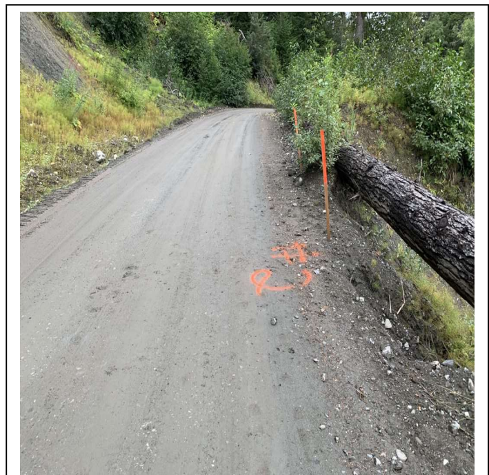
Site 4 GPS: 59.42115, -136.17052: Embankment #2, 260.7407 CY of native material sloped embankment, 8 FT long x 22 FT wide x 40 FT deep, high volume and high velocity surface water flooding scoured and washed out embankment.
