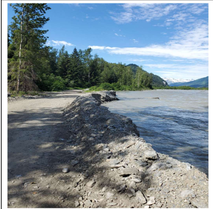
Riprap armor rock embankment, 2,449.7778 CY, 24–48-inch, 636 FT long x 13 FT wide x 8 FT deep, high volume and high velocity flooding washed out riprap embankment. Photo from applicant taken June 2021.
