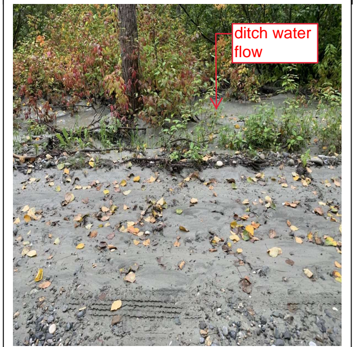
Perspective view of surface washout and normal current water flow through the ditches.
