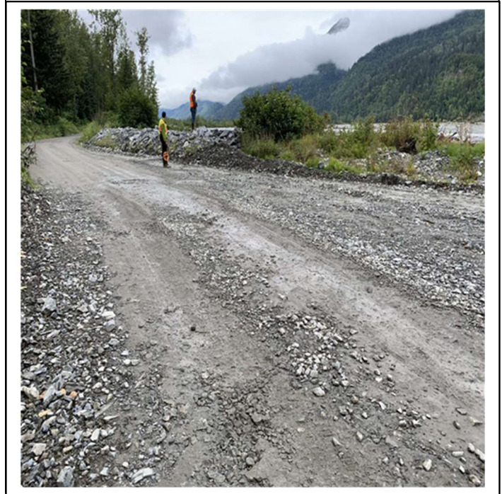
Site 9B GPS START: 59.41416, -136.08884 GPS END: 59.414363, -136.085552: Riprap armor rock embankment, 2,449.7778 CY of 24-48 inch minus, 636 FT long x 13 FT wide x 8 FT deep, high volume and high velocity flooding washed out riprap embankment.
