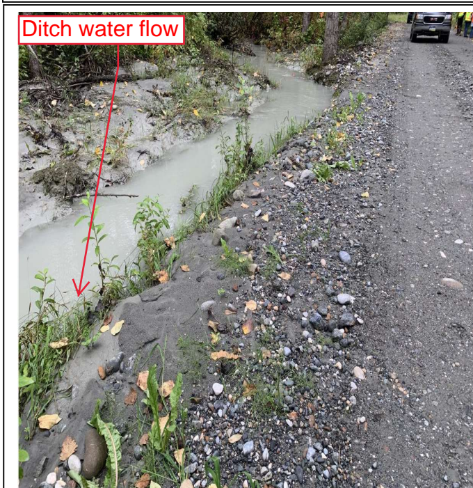
Site 2 GPS: 59.412354, -136.029592: Ditches, 7,626.6667 CY of native material drainage canals, 34,320 FT long x 3 FT wide x 2 FT deep, high volume and high velocity surface water flooding scoured and washed out ditches.
