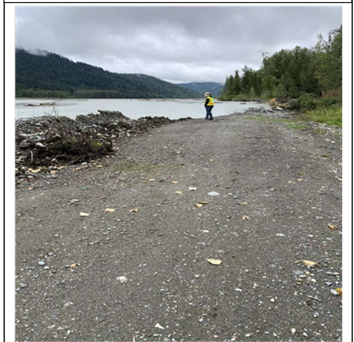
Site 9 GPS START: 59.41416, -136.08884 GPS END: 59.414363, -136.085552: Photo Taken August 26, 2021. Base, 471.1111 CY of native material, 636 FT long x 20 FT wide x 1 FT deep, high volume and high velocity surface water flooding washed out base.
