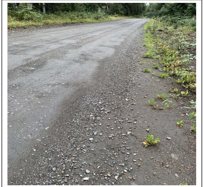
Site 1 GPS: 59.412354, -136.029592: Surface, 10,755.5556 CY of D1, 26,400 FT long x 22 FT wide x 0.5 FT deep, high volume and high velocity surface water flooding washed out road surface. Perspective view northwest.
