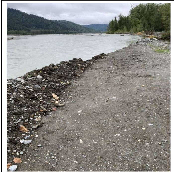
Site 9 GPS START: 59.41416, -136.08884 GPS END: 59.414363, -136.085552: Photo Taken August 26, 2021. Base, 471.1111 CY of native material, 636 FT long x 20 FT wide x 1 FT deep, high volume and high velocity surface water flooding washed out base
