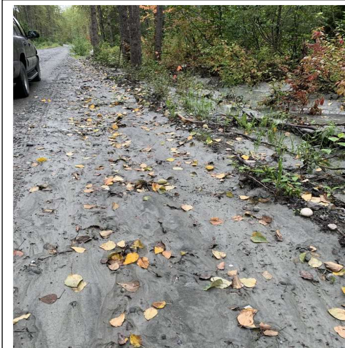
High volume and high velocity surface water flooding washed out 10,755.5556 CY of D1, 26,400 FT long x 22 FT wide x 0.5 FT deep of road surface.
