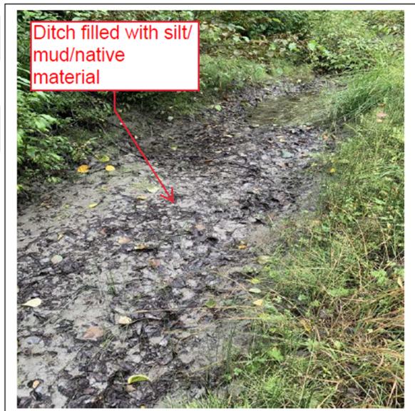
Figure 2: A typical location on Porcupine Trail Road showing vegetation encroachment on roadway shoulders and existing berms (the result of blading/grading maintenance) preventing drainage of storm water off roadway and/or to adjoining ditches, taken 6/7/2023 prior to Applicant's Phase 1 work. Source – Garret Gladsjo, proHNS.
