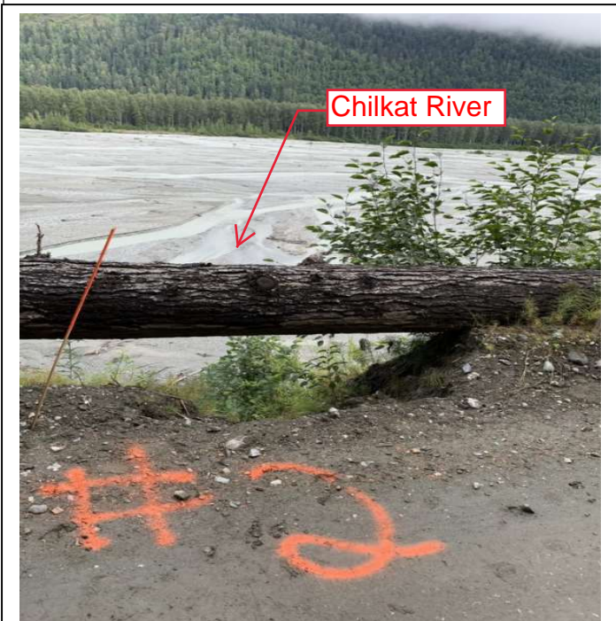
Site 4 GPS: 59.42115, -136.17052: Embankment #2, 260.7407 CY of native material sloped embankment, 8 FT long x 22 FT wide x 40 FT deep, high volume and high velocity surface water flooding scoured and washed out embankment.
