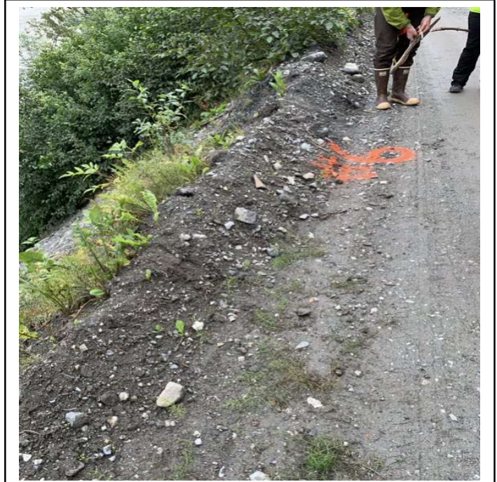
Site 8 GPS: 59.421193, -136.168441. Embankment, 1,356.6667 CY of native material sloped embankment, 30 FT long x 33 FT wide x 37 FT deep, high volume and high velocity surface water flooding scoured and washed out embankment.
