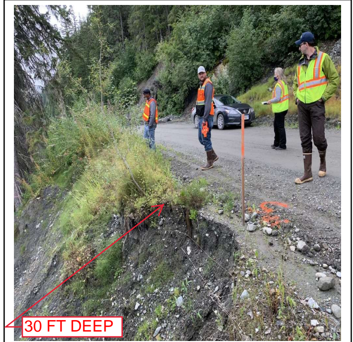
Site 7 GPS: 59.421530, -136.169010: Embankment #5, 1,111.1111 CY of native material sloped embankment, 20 FT long x 50 FT wide x 30 FT deep, high volume and high velocity surface water flooding scoured and washed out embankment.
