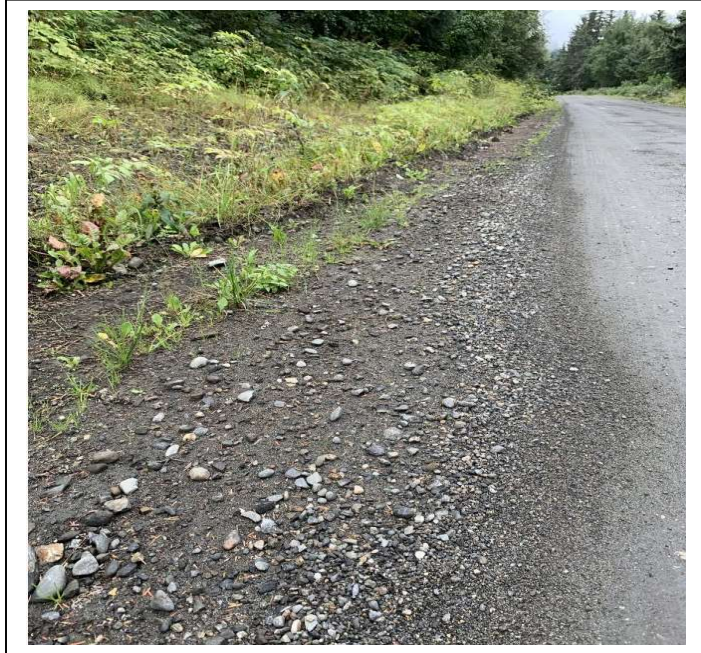
Site 1 GPS: 59.412354, -136.029592: Surface, 10,755.5556 CY of D1, 26,400 FT long x 22 FT wide x 0.5 FT deep, high volume and high velocity surface water flooding washed out road surface. Perspective view northwest.
