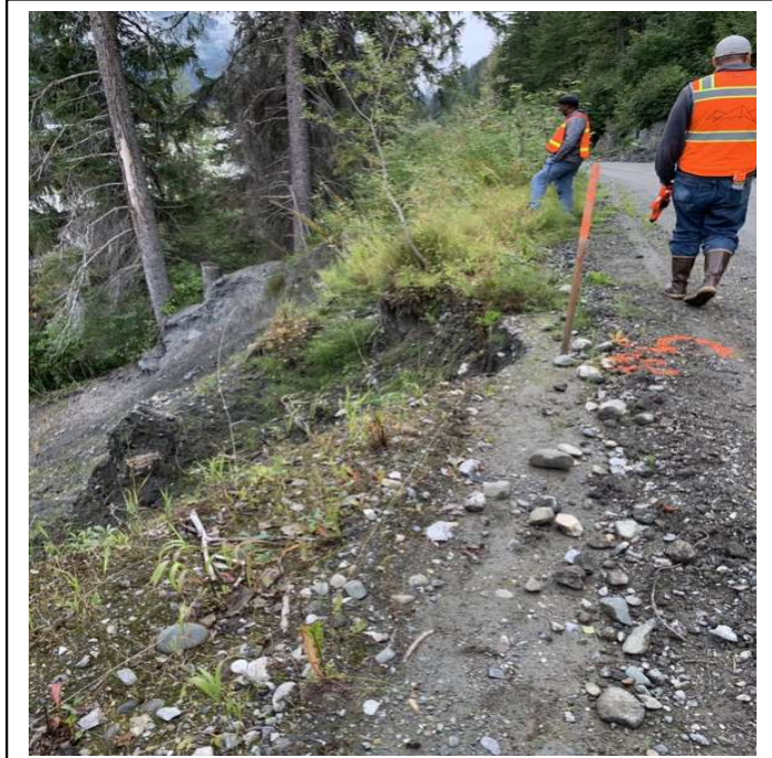
Site 7 GPS: 59.421530, -136.169010: Embankment #5, 1,111.1111 CY of native material sloped embankment, 20 FT long x 50 FT wide x 30 FT deep, high volume and high velocity surface water flooding scoured and washed out embankment.
