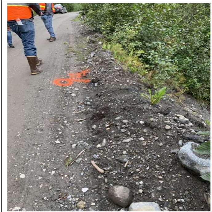
Site 8 GPS: 59.421193, -136.168441. Embankment, 1,356.6667 CY of native material sloped embankment, 30 FT long x 33 FT wide x 37 FT deep, high volume and high velocity surface water flooding scoured and washed out embankment.
