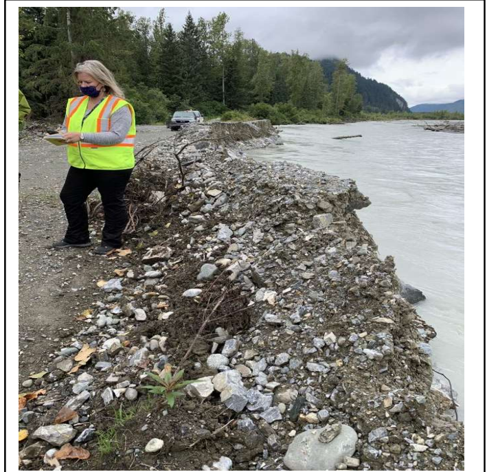
Riprap armor rock embankment, 2,449.7778 CY, 24-48 inch, 636 FT long x 13 FT wide x 8 FT deep, high volume and high velocity flooding washed out riprap embankment. Photo taken August 26, 2021
