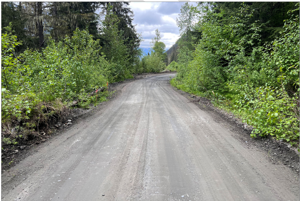
Figure 1: A typical location of vegetation encroachment on roadway shoulders and in ditches on Porcupine Trail Road, taken 6/7/2023 prior to Applicant’s Phase 1 work. Source – Garret Gladsjo, proHNS.
