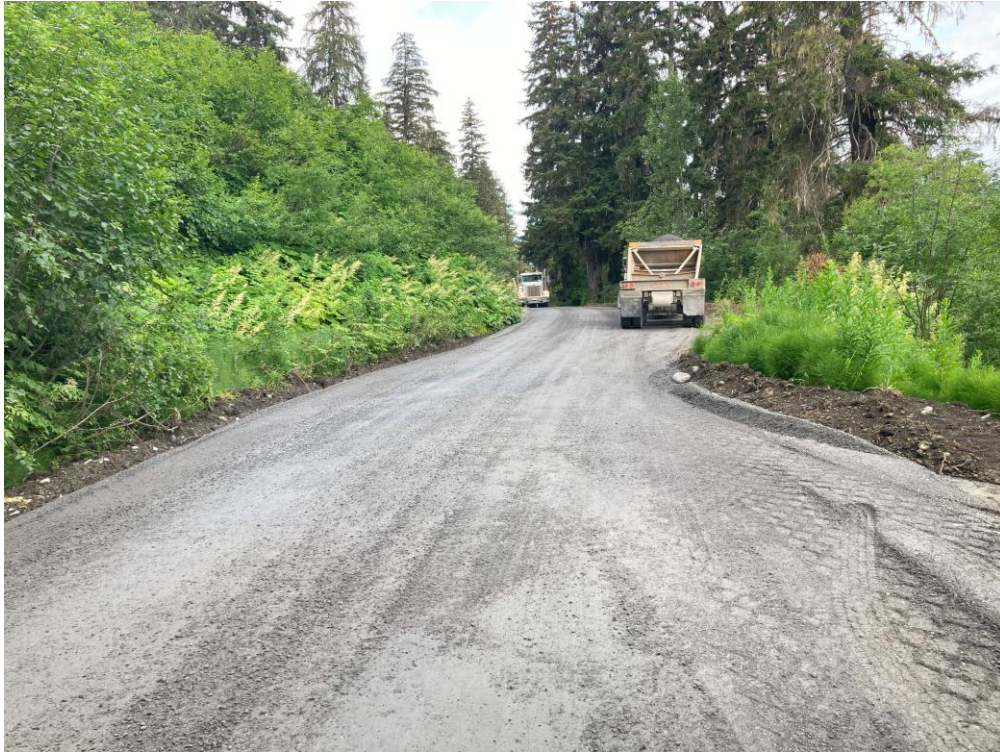
5.9 mile from B□P Calcium Chloride material haul
