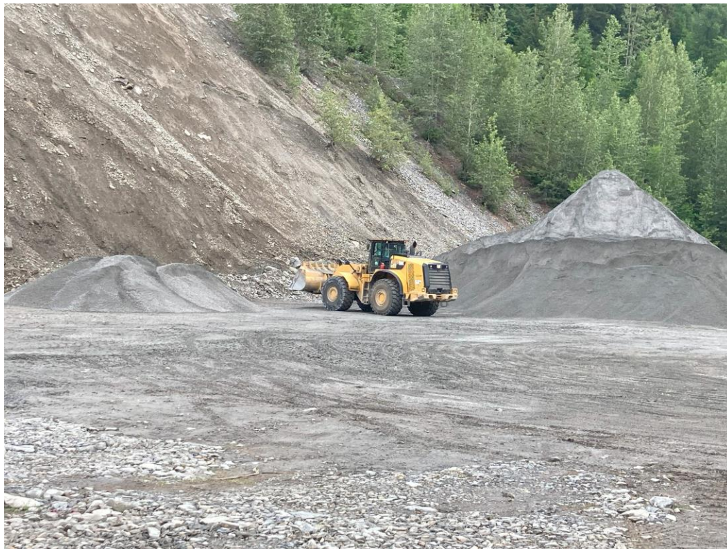
10 am E1 stockpile with Calcium Chloride
