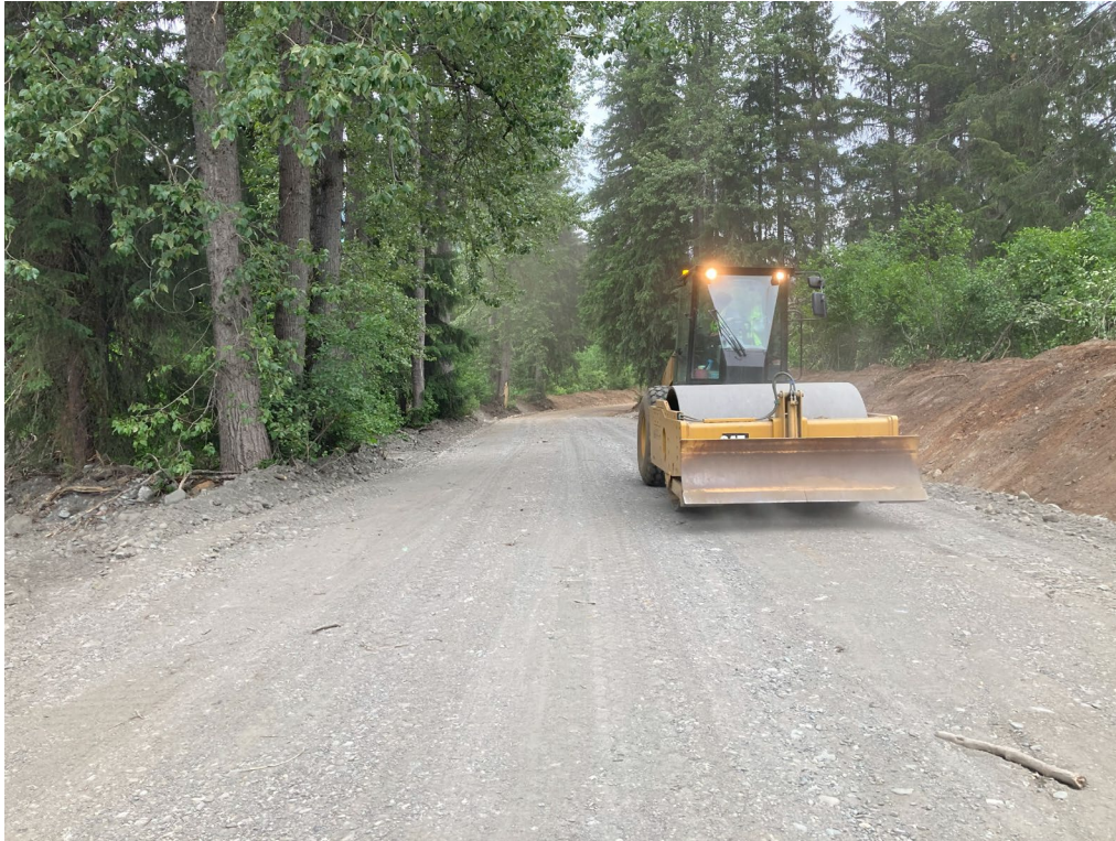
Last day of Reconditioning, Roadbed and Shoulders
