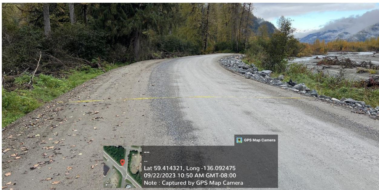
Figure C.7 – Cross section of third-party work site 3 fill area on Porcupine Trail Road, outside of Phase I work limits. Edge of shoulder to edge of shoulder width is 28' at this location (including pullout), and width to outside edges of travel lanes (driving surface) is 15.7'. Third-party work at this site was placement of 3' fill and some riprap above ordinary high water – no gravel surfacing materials were placed. Fill was placed within the limits of the existing roadway corridor shoulders/berms. Photos of measurements can be provided upon request.
