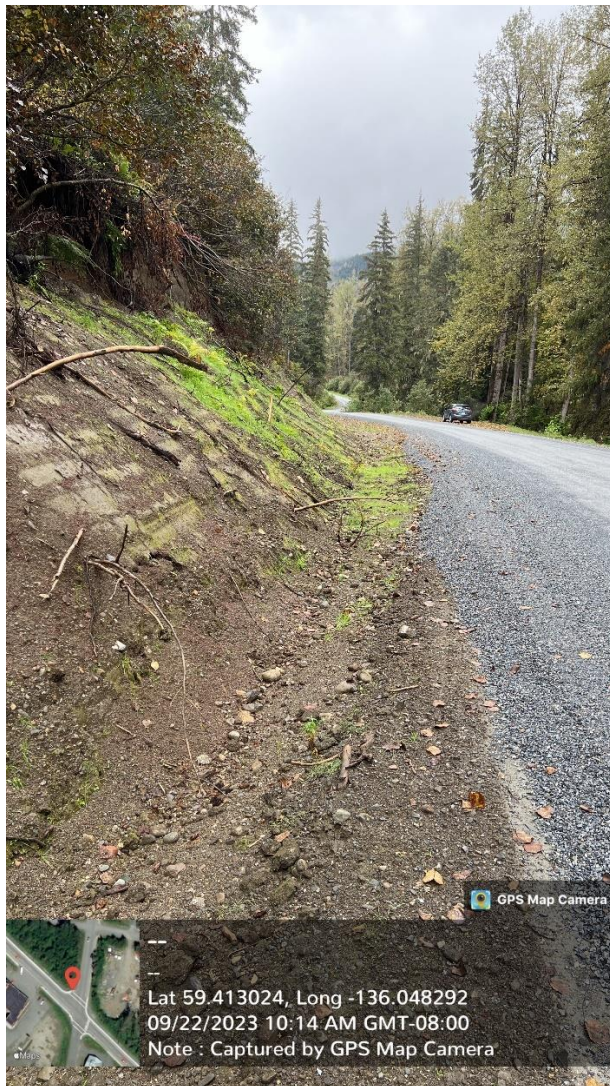
Figures G.3 (LT) and G.4 (RT) – Source of Third-Party work fill material for sites 1-3. Contractor sourced native material for fill, with approval from Alaska DNR, from existing slope adjacent to Porcupine Trail Road near Milepost 1. No other material was sourced from this location, which is within the roadway right-of-way.
