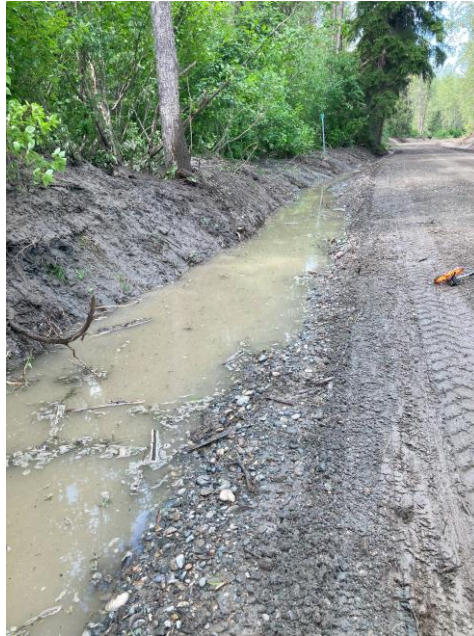
2 mi. marker ditch line with water
