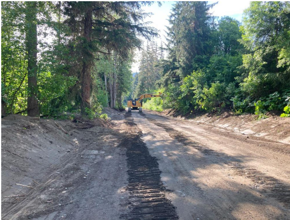
Jeff/335 left ditch line, working back towards Ron.
