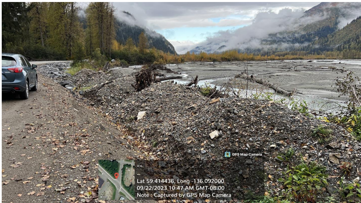
Figure H.6 – Berm on right was placed in 2022 as described in FH22-I-0090. This is the same location as 2023 Third-Party Work Site 3. Third-party work placed 3' of road fill up against backside of berm placed in 2022. Riprap placement above ordinary high water by third-party work in 2023 can be seen beyond front of vehicle in this photo (refer to Figures C.8 and C.9).
