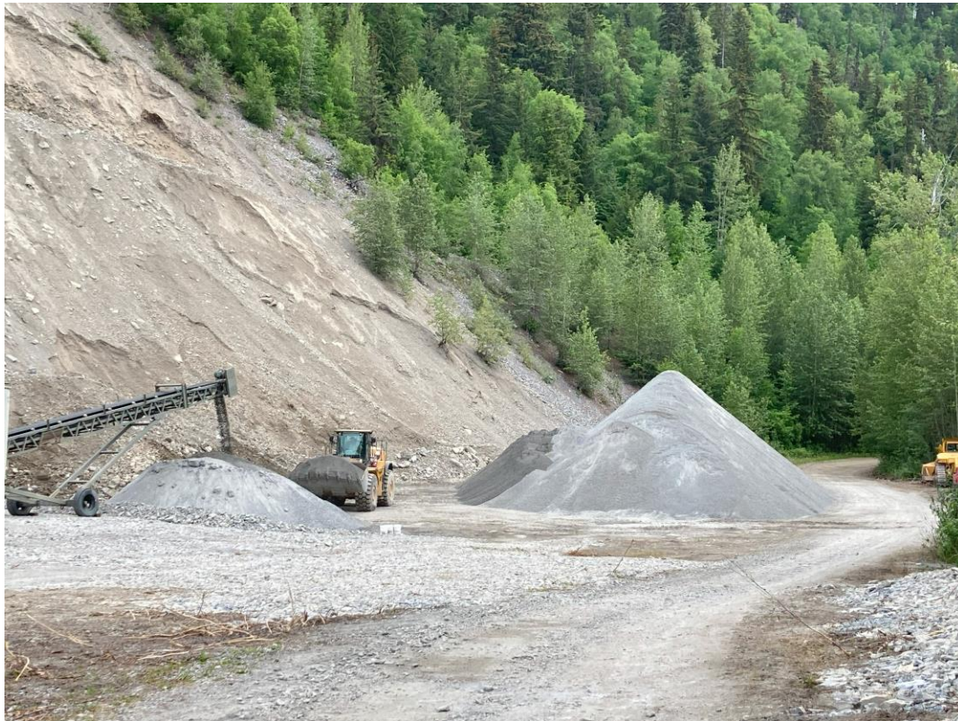
E1 stockpile. 3 samples taken/day off the belt
