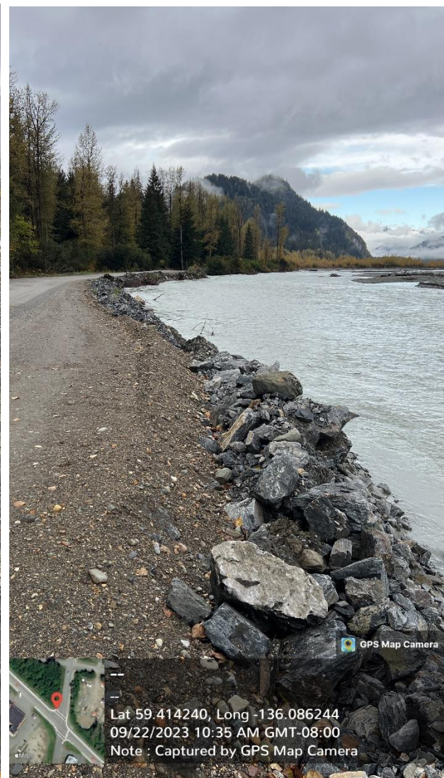
Figures H.3 (LT) and H.4 (RT) – Berms in background of photo at left, and riprap in photo at right, were placed in 2022 as described in FH22-I-0090. This is the same location as 2023 Third-Party Work Site 2. Third-party work placed 3' of road fill up against backside of riprap and berms placed in 2022. Figure H.3 on left shows elevation of existing road grade at backside of berms prior to 3' fill placement.
