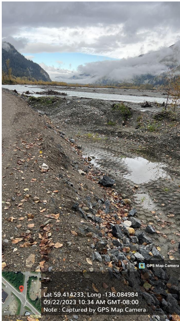
Figures H.3 (LT) and H.4 (RT) – Berms in background of photo at left, and riprap in photo at right, were placed in 2022 as described in FH22-I-0090. This is the same location as 2023 Third-Party Work Site 2. Third-party work placed 3' of road fill up against backside of riprap and berms placed in 2022. Figure H.3 on left shows elevation of existing road grade at backside of berms prior to 3' fill placement.
