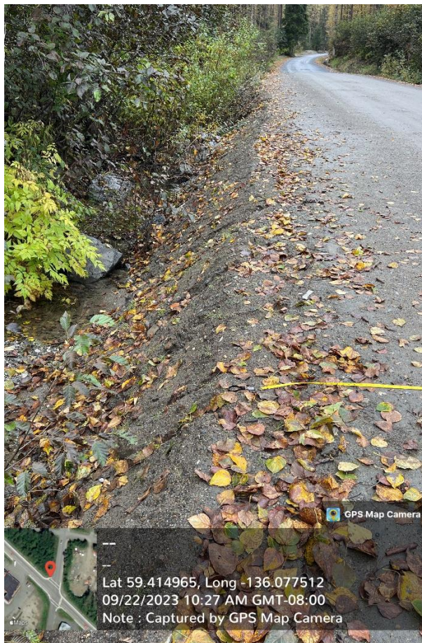
Figures C.4 (LT) and C.5 (RT) – 1:1 sloped embankment for 3’ fill at third-party work site 1 fill area. Note the toe of fill has been placed at the edge of the existing roadway, leaving the existing ditches on the left and right side of photos untouched.
