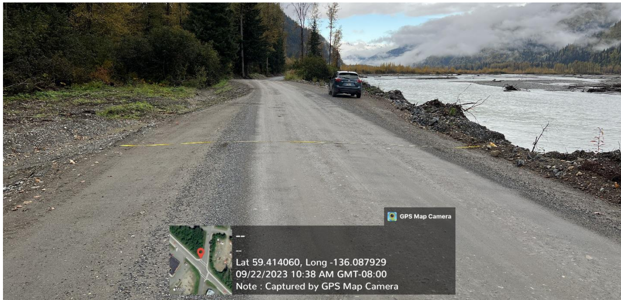
Figure C.6 – Cross section of third-party work site 2 fill area on Porcupine Trail Road, outside of Phase I work limits. Edge of shoulder to edge of shoulder width is 28' at this location (including pullout), and width to outside edges of travel lanes (driving surface) is 16'. Third-party work at this site was placement of 3' fill only – no gravel surfacing or riprap materials were placed. Fill was placed within the limits of the existing roadway corridor shoulders/berms. Photos of measurements can be provided upon request.
