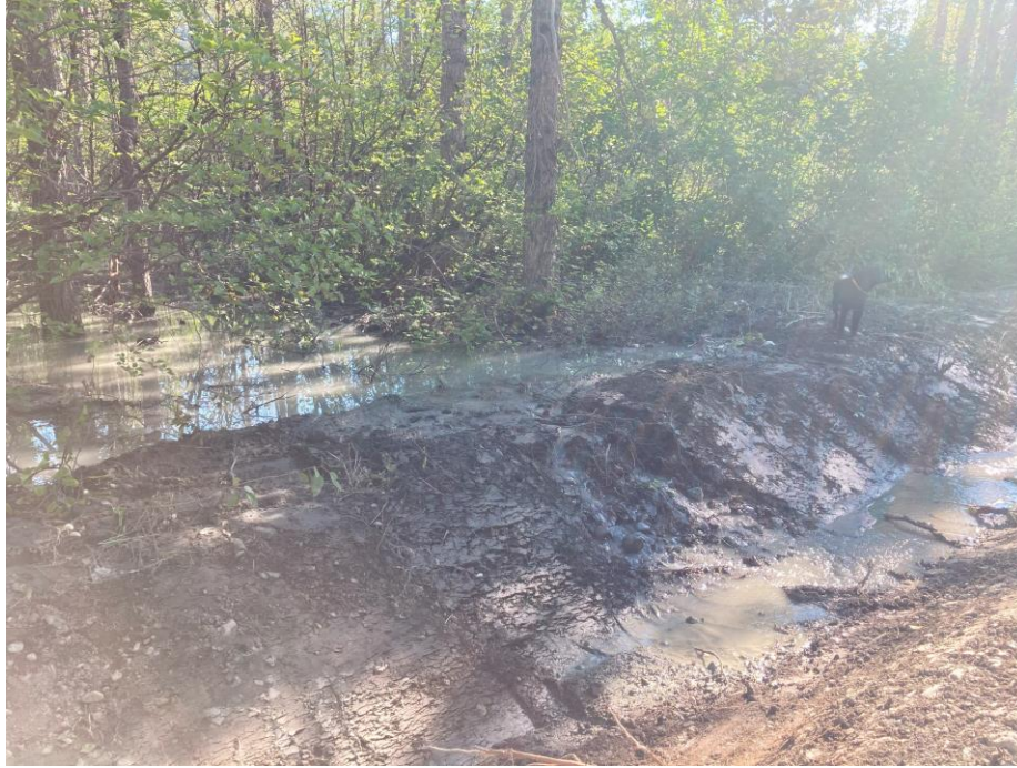
Water coming into the cleaned ditches
