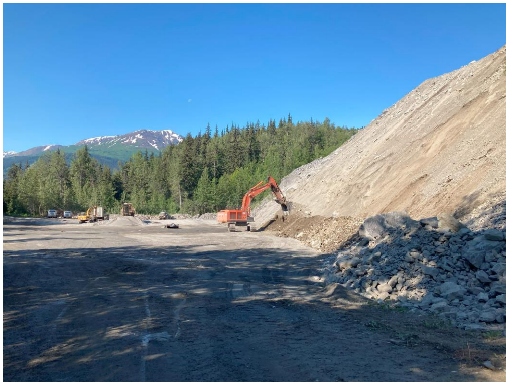
Pit final clean up.
