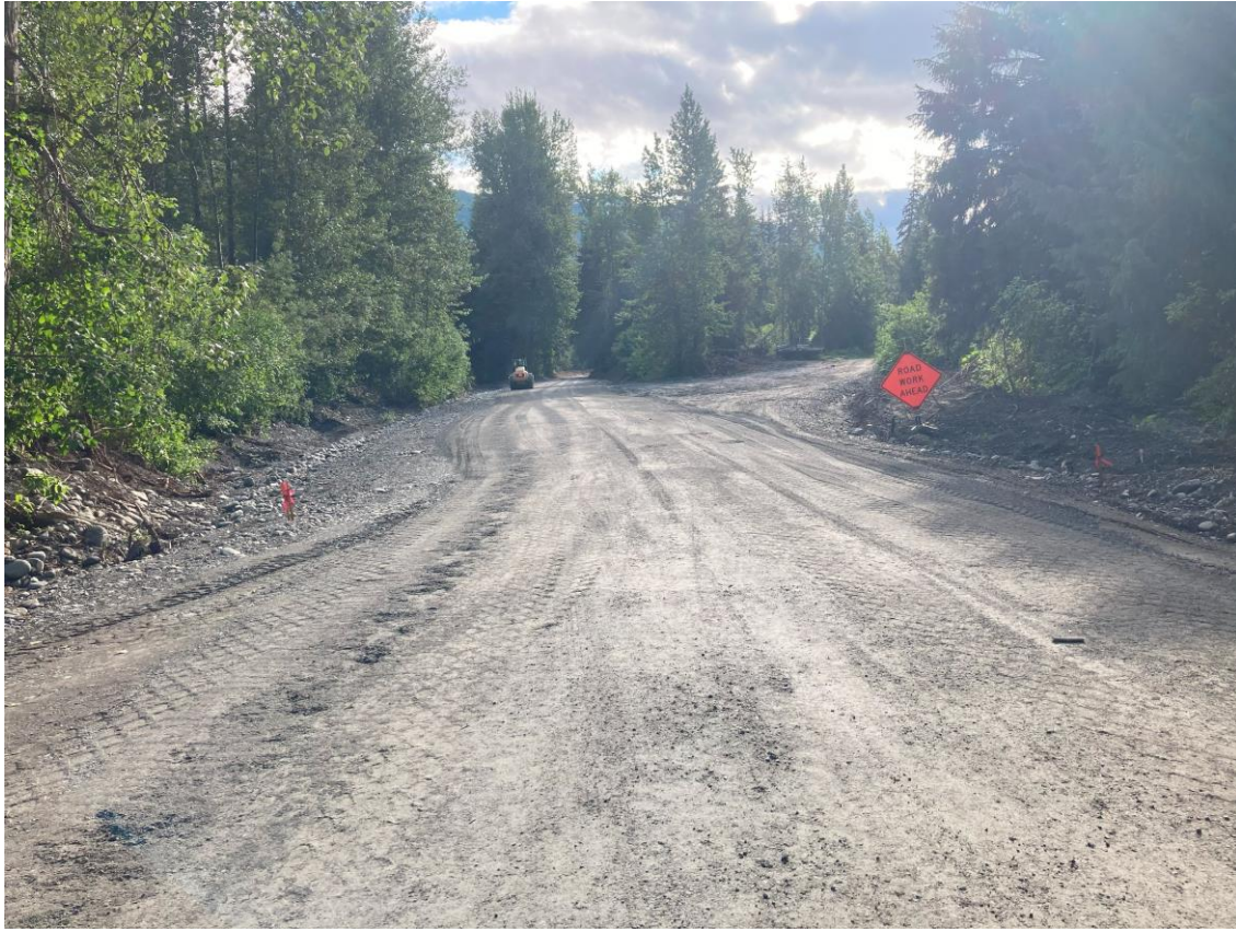
Cat 663E Roller finishing up the first lift of E1
