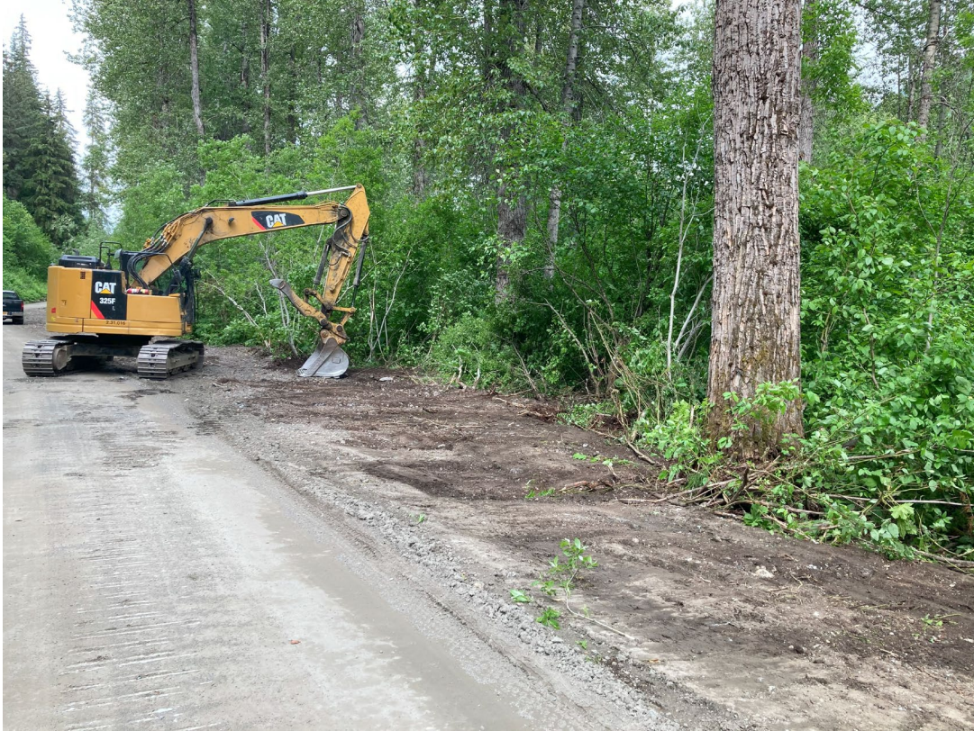
Ron/325F 3 rd Segment
