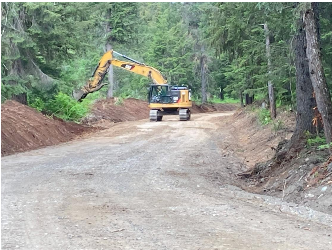
Last day of Reconditioning of Ditches
