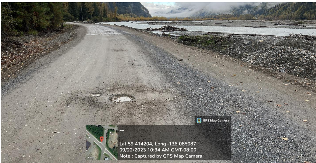
Figure H.2 – Berm on right was placed in 2022 as described in FH22-I-0090. This is the same location as 2023 Third-Party Work Site 2. Third-party work placed 3’ of road fill up against backside of berm placed in 2022.
