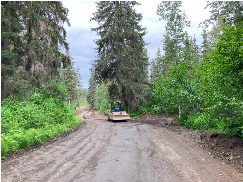
Road Reconditioning continues. 6.5 mile from B1P
