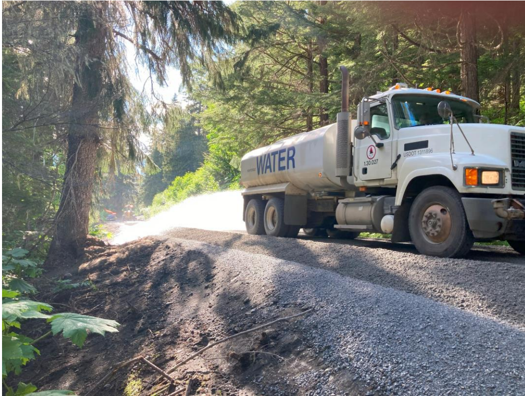
Water truck heavily waters the E1 with Calcium Chloride
