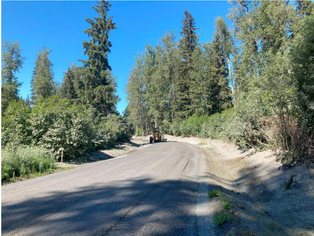
Finishing up haul 0.7 mile from BOP
