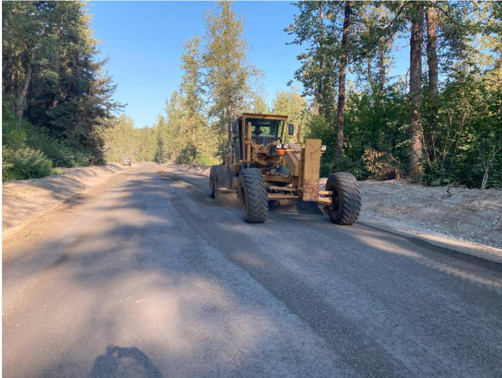
14 Grader finish grading 1.3 miles from B P
