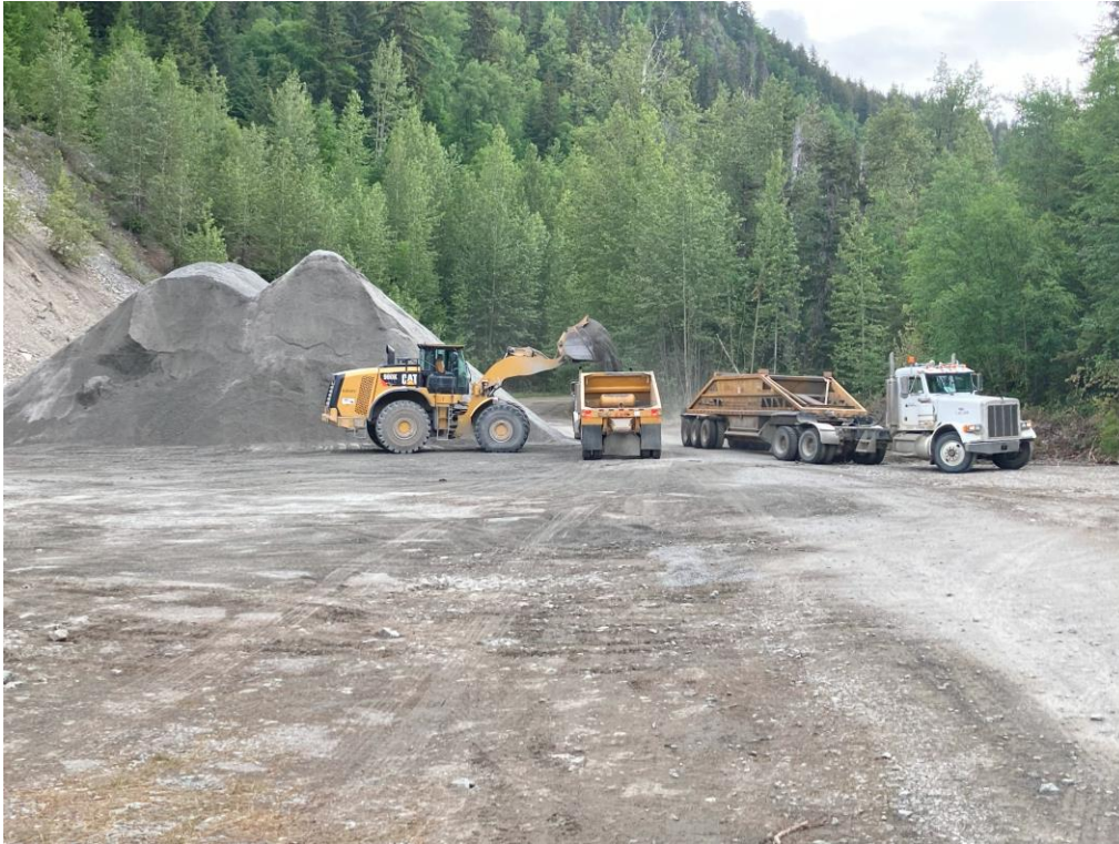
Pit today. Teri loading trucks
