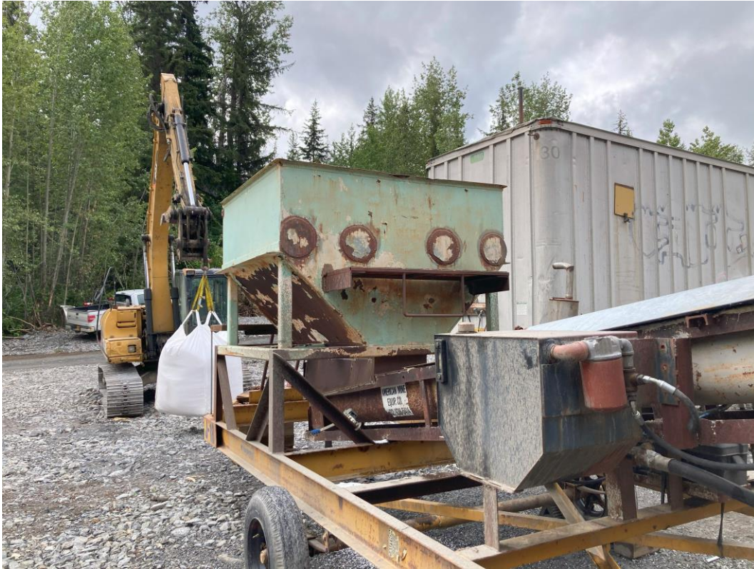
Calcium Chloride added to belt through screw feeder
