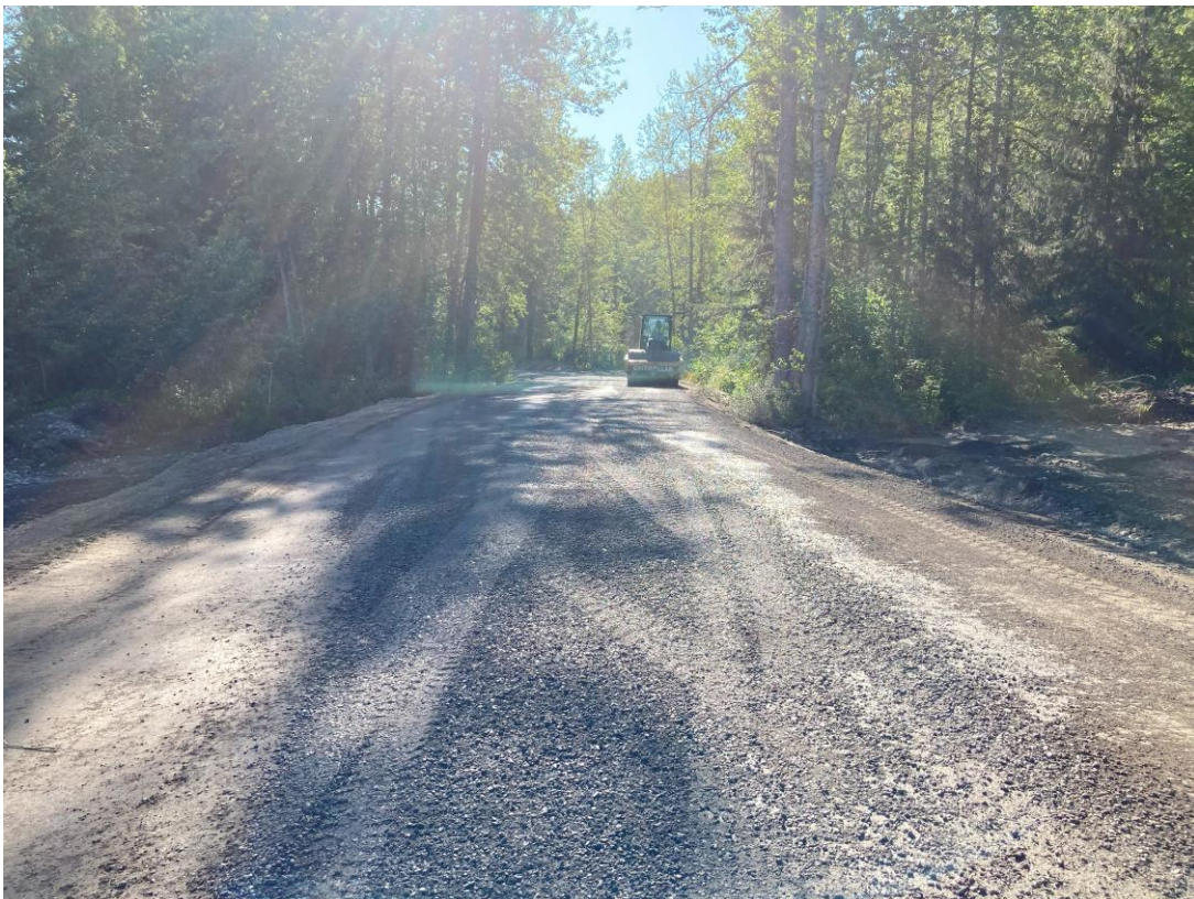
Roller working with the laydown crew 2.3 miles from BOP
