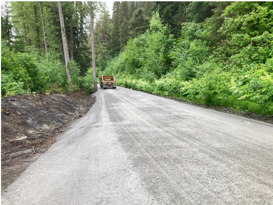
Project ditches, roadway
