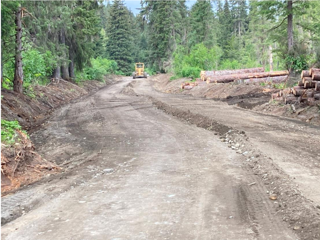
14 Grader at 6.5 from B P, Road Reconditioning
