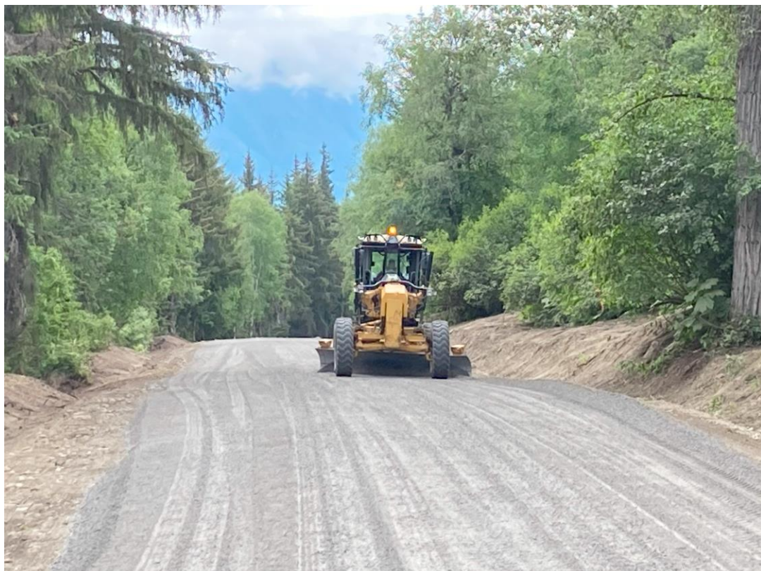
SERB Grader/Steiner placing E1 material
