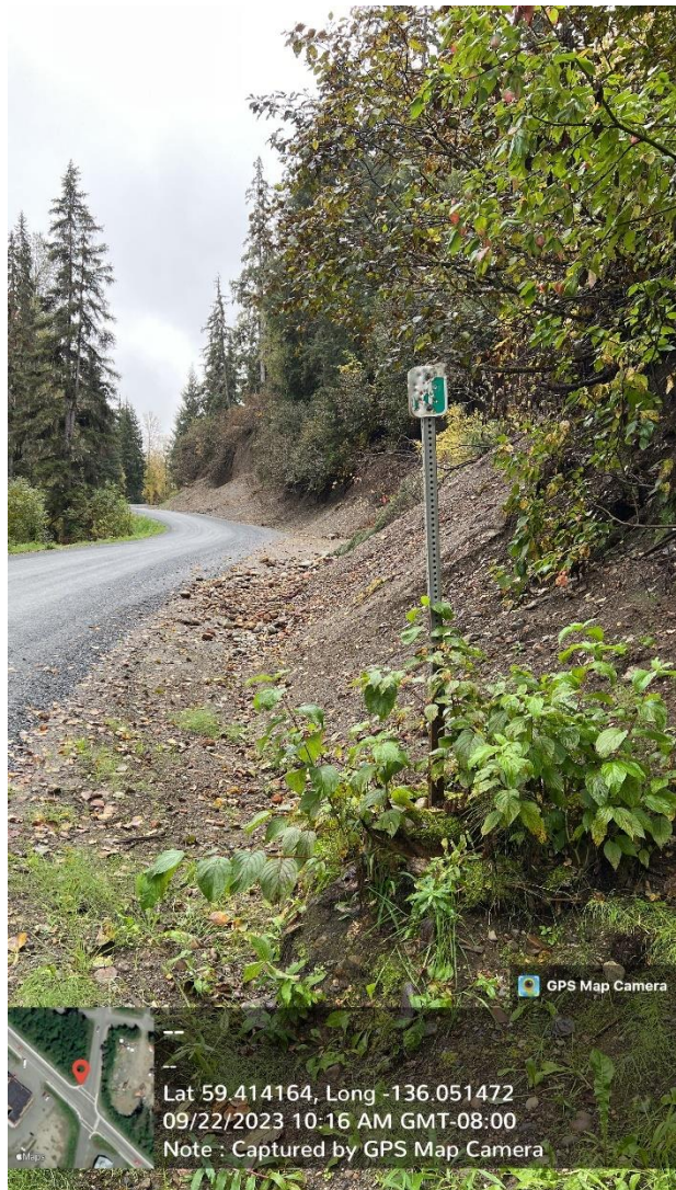
Figures G.3 (LT) and G.4 (RT) – Source of Third-Party work fill material for sites 1-3. Contractor sourced native material for fill, with approval from Alaska DNR, from existing slope adjacent to Porcupine Trail Road near Milepost 1. No other material was sourced from this location, which is within the roadway right-of-way.
