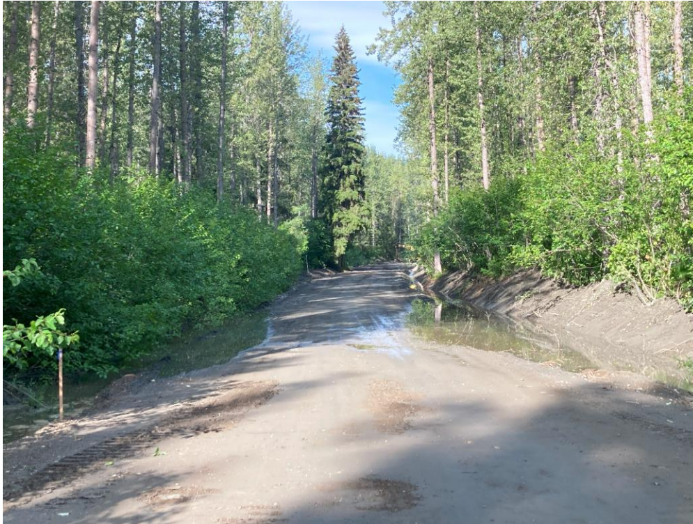
The one area today that overflow exceeded ditch line
