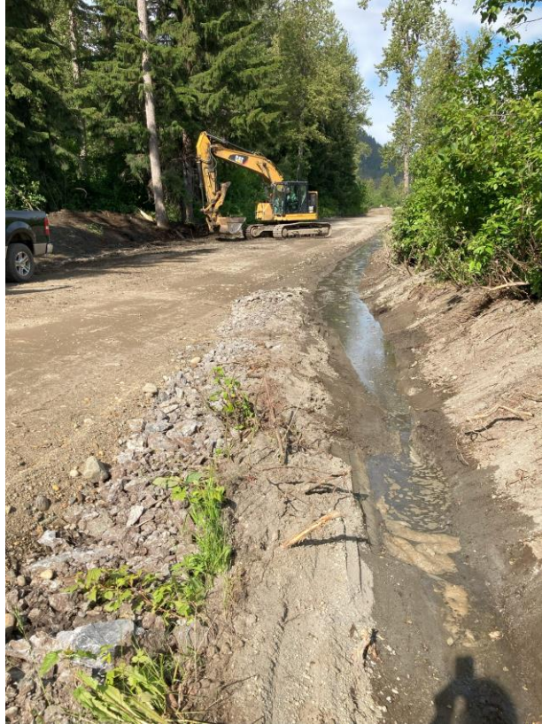
Water level down in ditch, from yesterday
