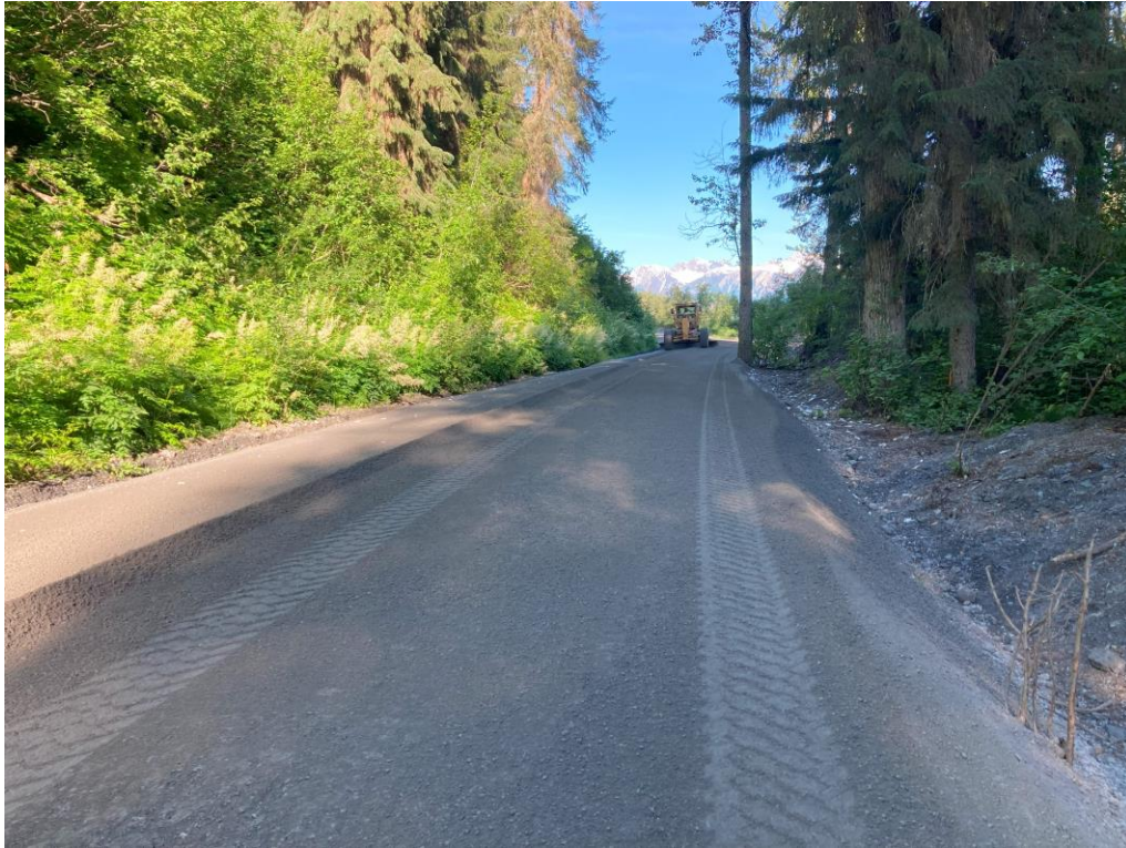
14 Grader finish blading 4.5 miles from B-P
