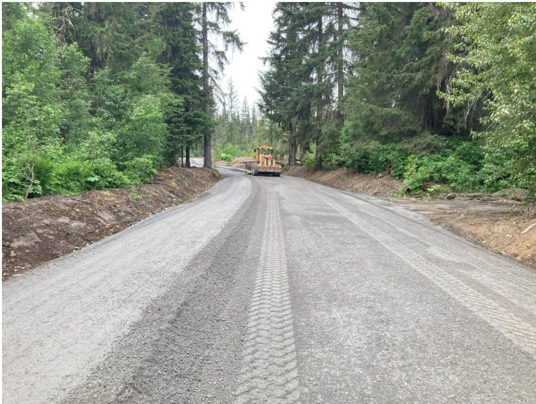
Cat 14G Grader started finish grading. 6.3 miles from B□P
