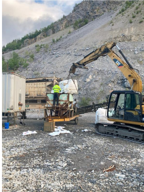
loading the Calcium Chloride in to screw feeder
