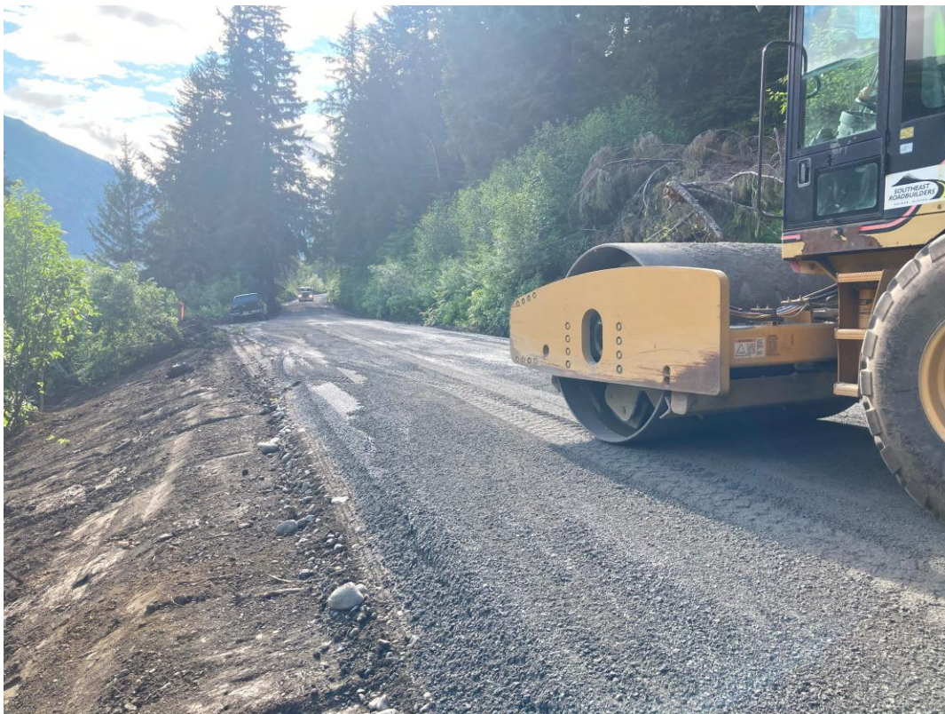
Roller working with the 14G Grader.
