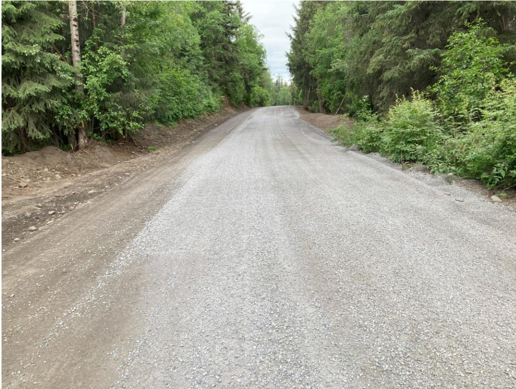
Two loads of E1 placed on project yesterday
