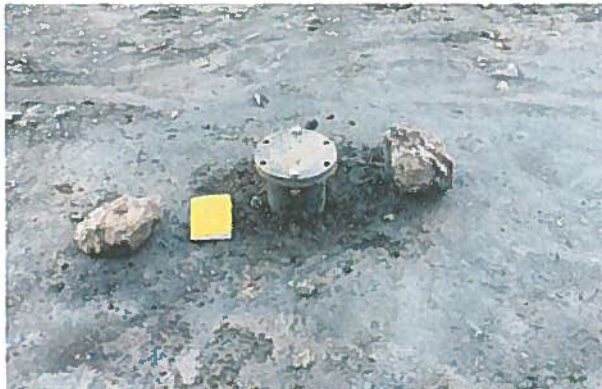
Photo 2 Example of Environmental Monitoring Well (Palmer Project, 2021)
