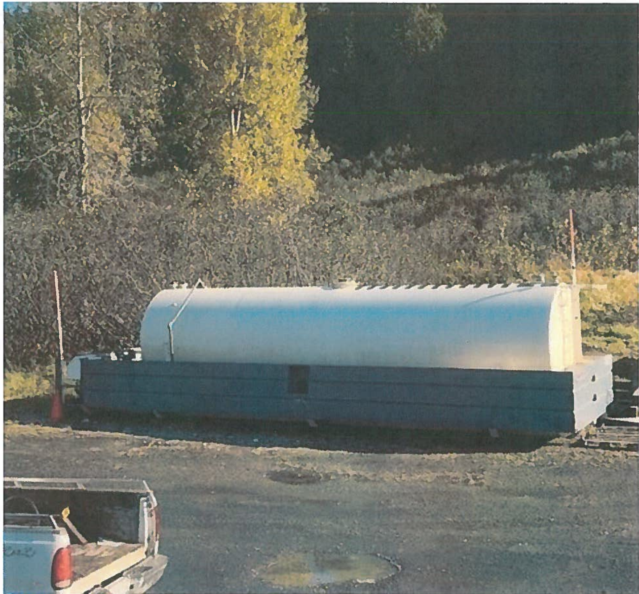
Photo 2: 10,000-gallon fuel tank at Glacier Creek Laydown (added in 2018). Note that this tank is currently not in use and is staged for Phase 2 Plan of Operation (Photo: Oct 2021).
