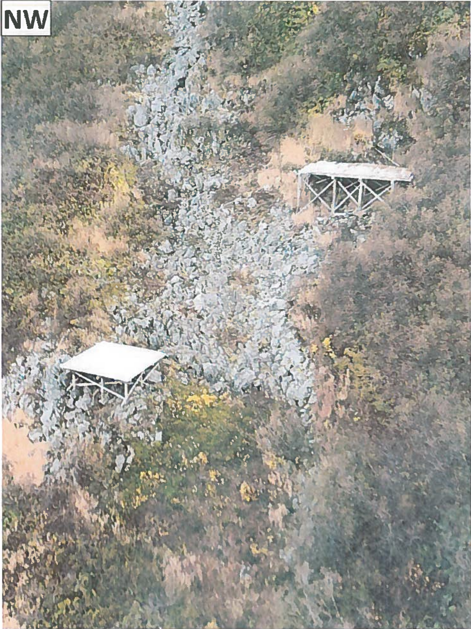
Photo 24: Aerial view of U6 Drill/Pump Pad (upper), built in 2014. U6 Pump was used to source water for 2022 B-Lo drill pad holes. Pad retains decking and remains unreclaimed for potential future use.
