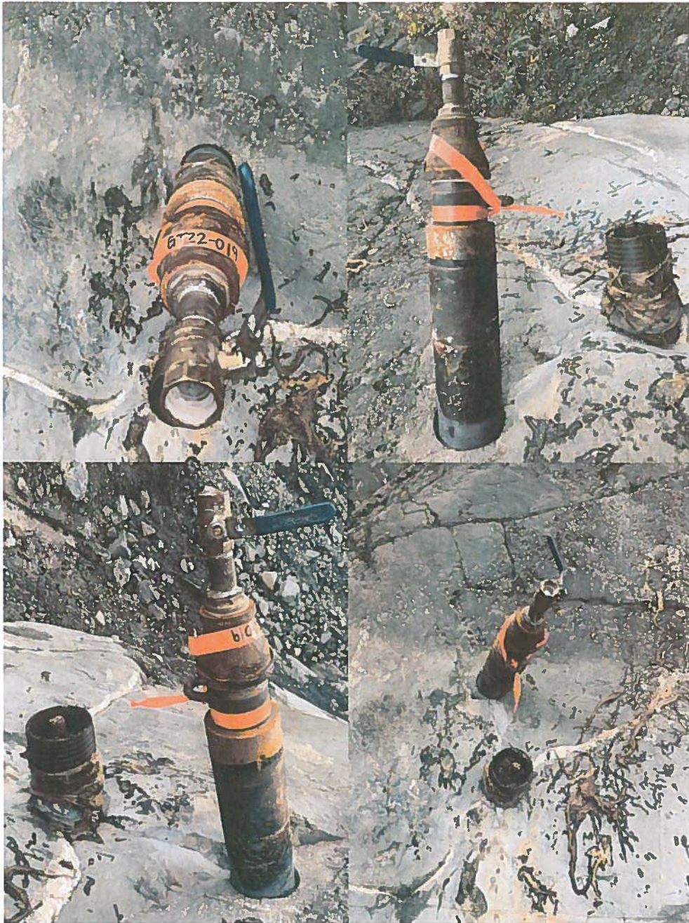
Photo 10: Wormhole Pad diamond drill hole GT22-019 is capped using a standpipe with valve.
