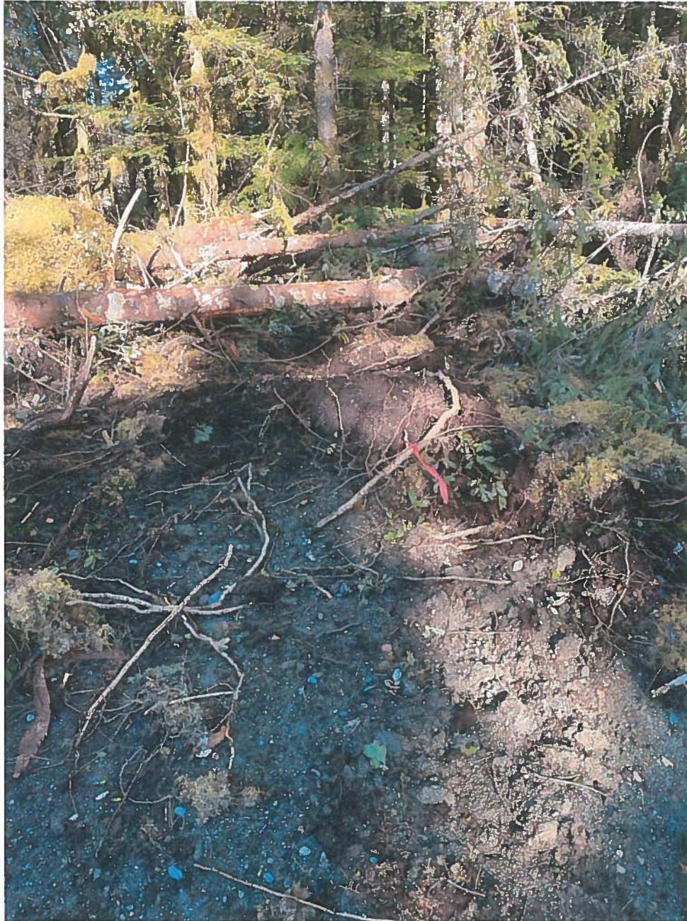
FIGURE 4.3 EXAMPLE OF DRILL PAD SITE PREP. ORGANICS WILL BE STOCKPILED FOR RECLAMATION POST DRILLING. EROSION AND UNDUE DEGRADATION WILL BE MITIGATED WITH ACTIVE SITE MANAGEMENT
