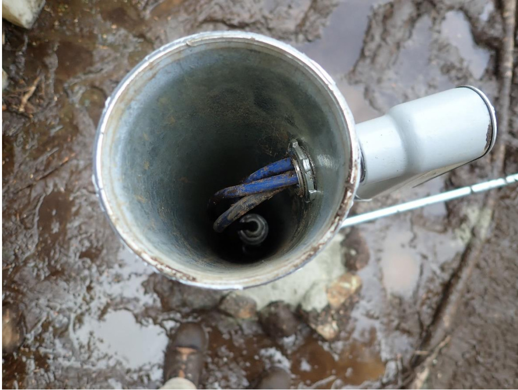
A: Typical monument completion with instrument cables routed
