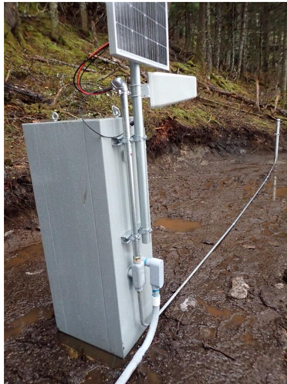
B: Base station installation at LT-6 (view looking west)
