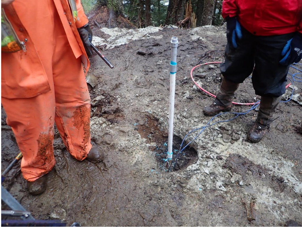
A: Typical PVC casing installation prior to SAAV installation
