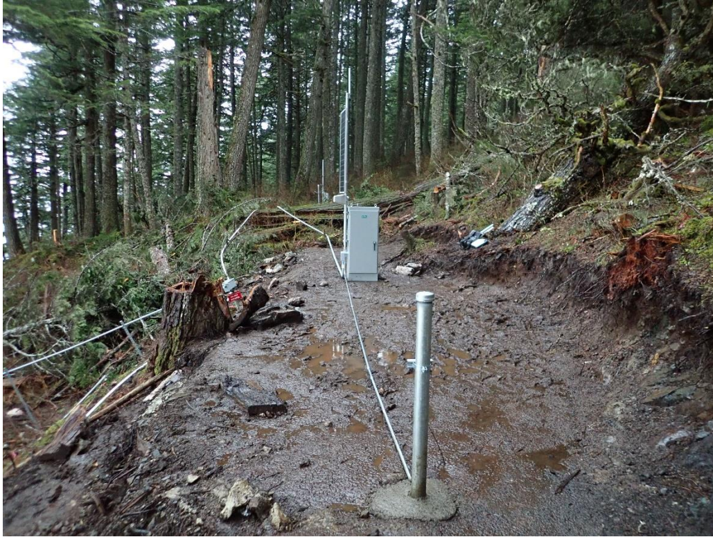
A: Base station installation at LT-6 (view looking east)
