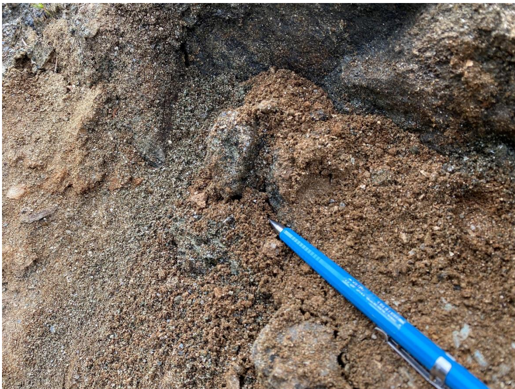
B: Colluvium 1 at elevation 620 feet on the West Soil Scarp.
