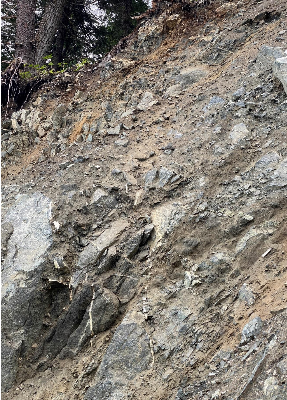
Colluvium 1 at elevation 670-680 on the West Soil Scarp.
