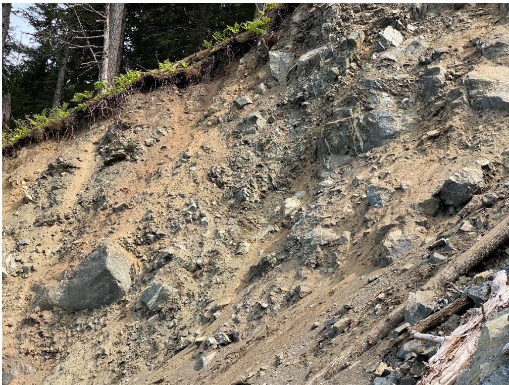
B: Colluvium 1 at elevation 650-680 on the West Soil Scarp.
