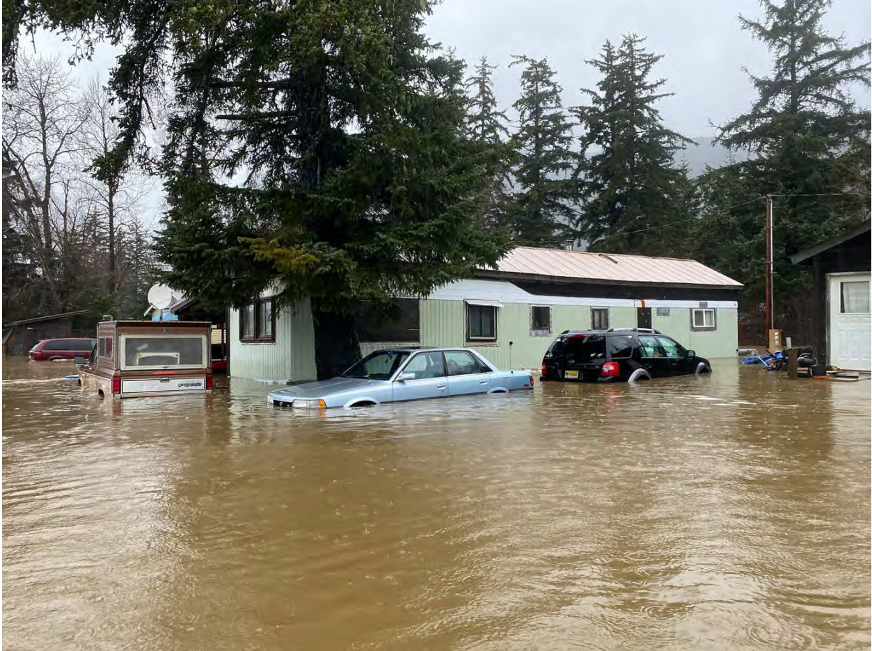
Figure 9. Floodwater in Haines, December 2020
