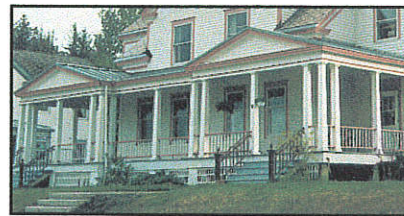
More ordinary porch has square balusters and railing and square posts.
