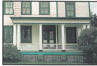
High "ranking" building with turned spindles and shaped railing on porch.
