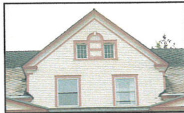
Most standard type of eaves. Returns w/capitols on top of corner boards.
