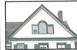
Most buildings in the entire fort have the same roof pitch. "Standard pitch" for the fort is 9:12.
