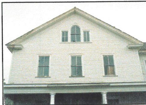
Deep soffits w/returns and built in gutters.
