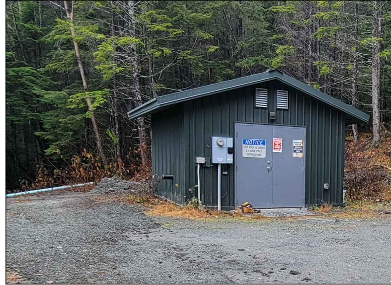
2 PHOTO - SERVICE EQUIPMENT E-202
