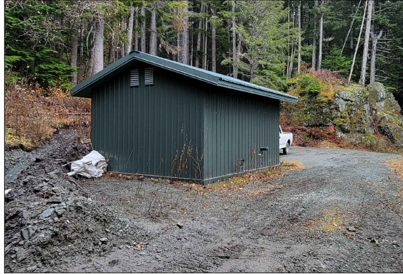
1 PHOTO - GENERATOR SITE E-202
