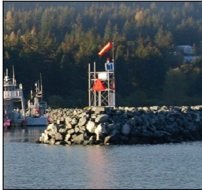
EXISTING NAV-AID STRUCTURE
