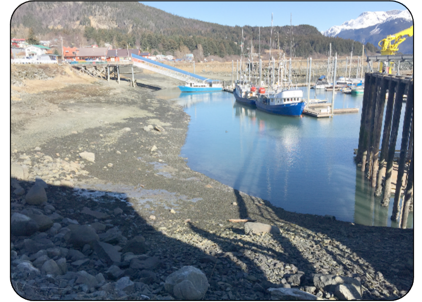
C INNER HARBOR DREDGE AREA LOOKING NORTH
