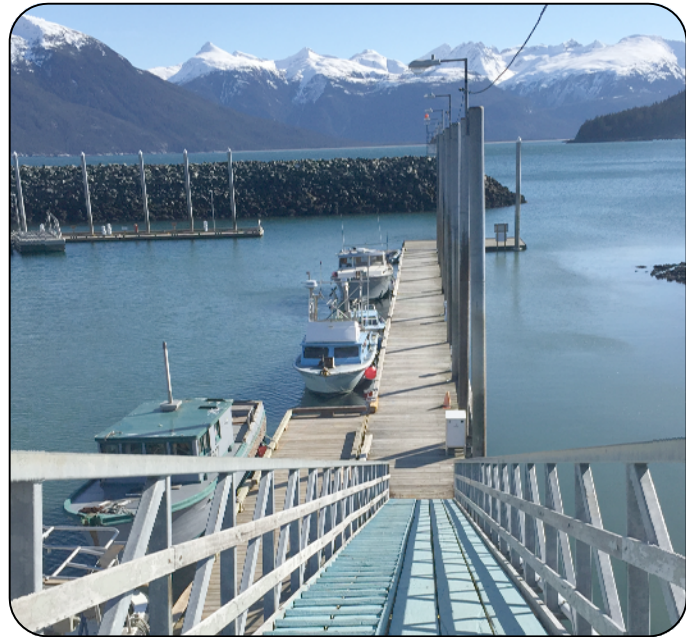
E TRANSIENT FLOAT PILES TO BE REPLACED EXISTING LIGHT FIXTURES TO BE SALVAGED AND REINSTALLED BY CONTRACTOR. POWER CABLE TO BE SALVAGED BY CONTRACTOR, POWER CABLE TO BE INSTALLED BY OWNER
