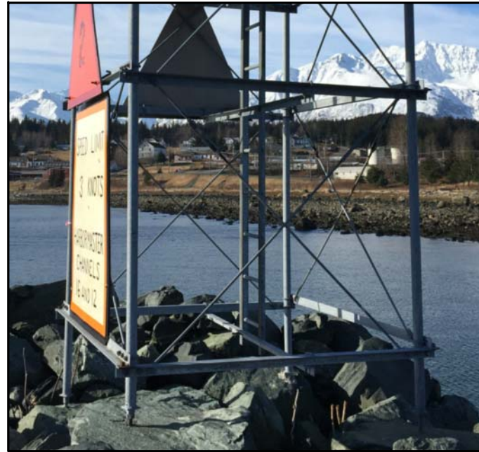
EXISTING NAV-AID FOUNDATION
