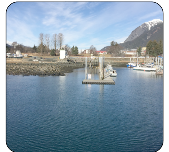
G DREDGE AREA LOOKING WEST AT TRANSIENT FLOAT
