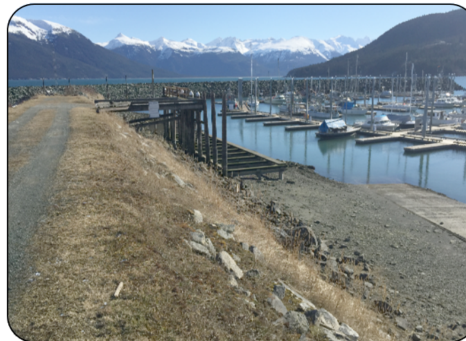
F DREDGE AREA INNER HARBOR LOOKING EAST
