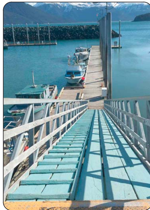
E TRANSIENT FLOAT PILES TO BE REPLACED EXISTING LIGHT FIXTURES TO BE SALVAGED AND REINSTALLED BY CONTRACTOR. POWER CABLE TO BE SALVAGED BY CONTRACTOR, POWER CABLE TO BE INSTALLED BY OWNER
