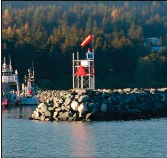
EXISTING NAV-AID STRUCTURE
