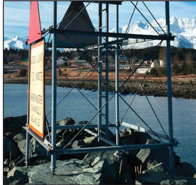
EXISTING NAV-AID FOUNDATION
