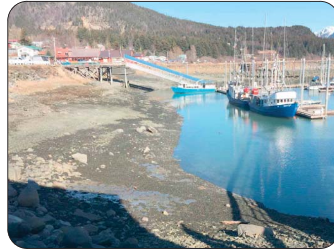
C INNER HARBOR DREDGE AREA LOOKING NORTH
