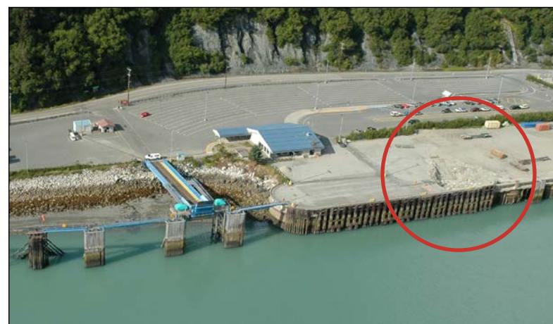
Figure 8: 2004 Collapse Near Alaska Marine Highway System Terminal
