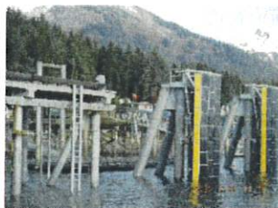
Tenakee Springs Ferry Terminal
