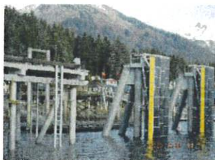
Tenakee Springs Ferry Terminal
