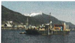
Offshore drilling at Gravina Freight Dock
