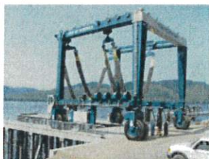
Hoonah Marine Industrial Center
