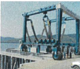
Hoonah Marine Industrial Center
