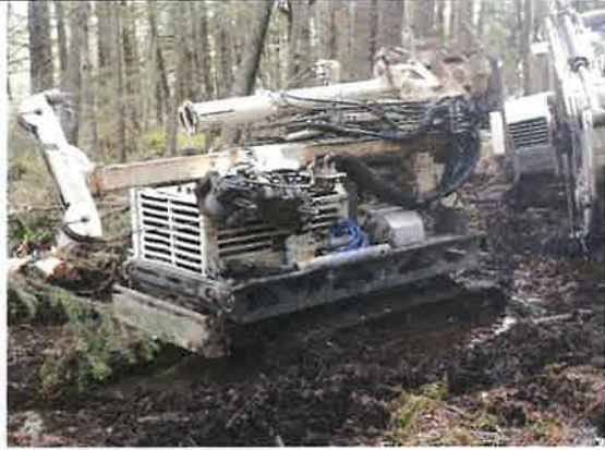
Photo 57: Geoprobe 6712 DT enroute to B-6
