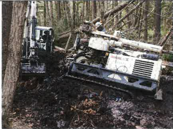
Photo 59: Excavating Geoprobe 6712 DT
