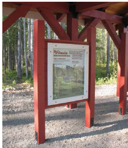
This option shows how a kiosk can be incorporated into structural elements or take on the character and use details from surrounding designs.
