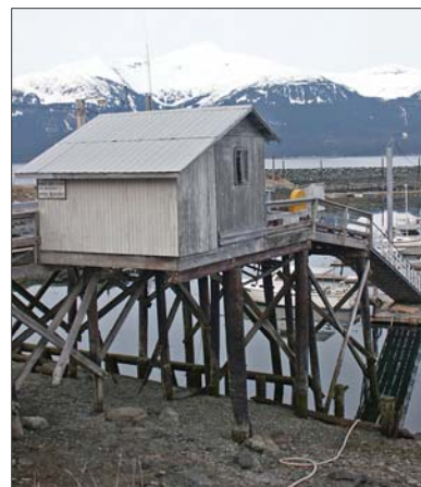
Haines Harbormaster Office
