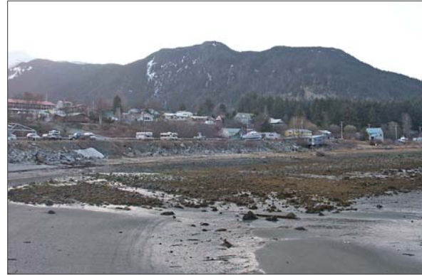
Area north of existing harbor: Harbor Expansion
